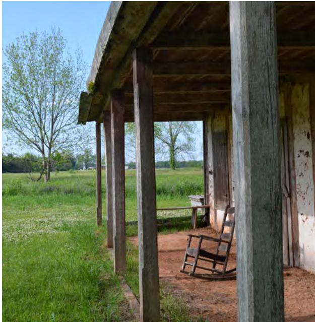
Left: The gutters on the house are causing decay of the framing. They should be removed and replaced with appropriate new gutters.
