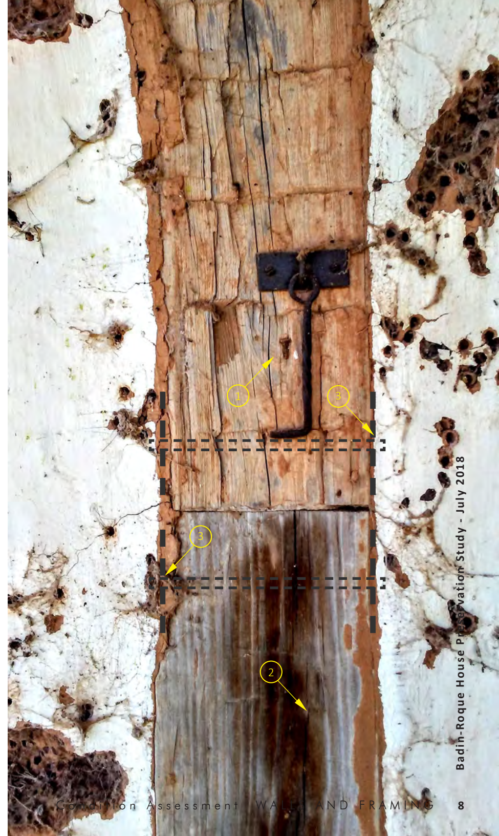
Right: A typical post splice. The upper part is original cypress, the lower part is c. 1990 southern pine.
