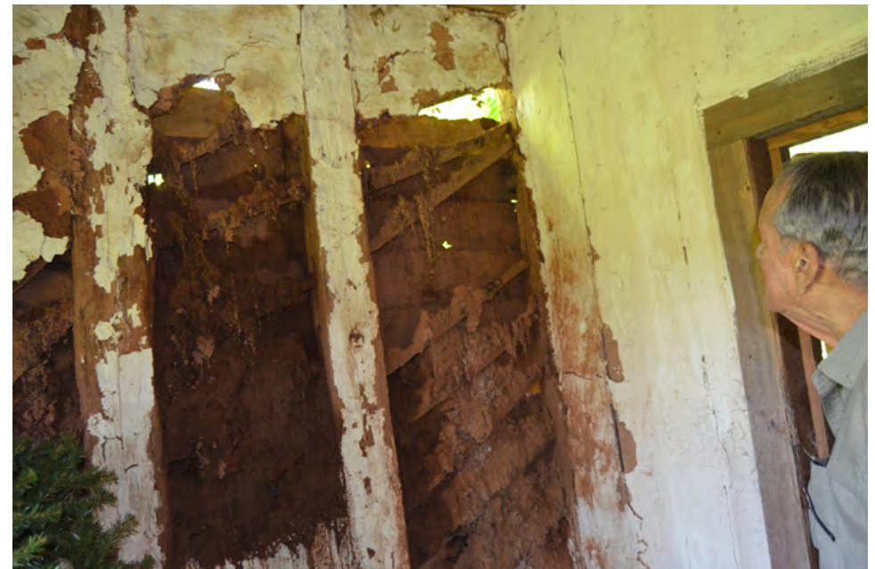
Right: Deterioration of the posts and bousillage walls in the rear of Room "D". These posts must be fully replaced.
