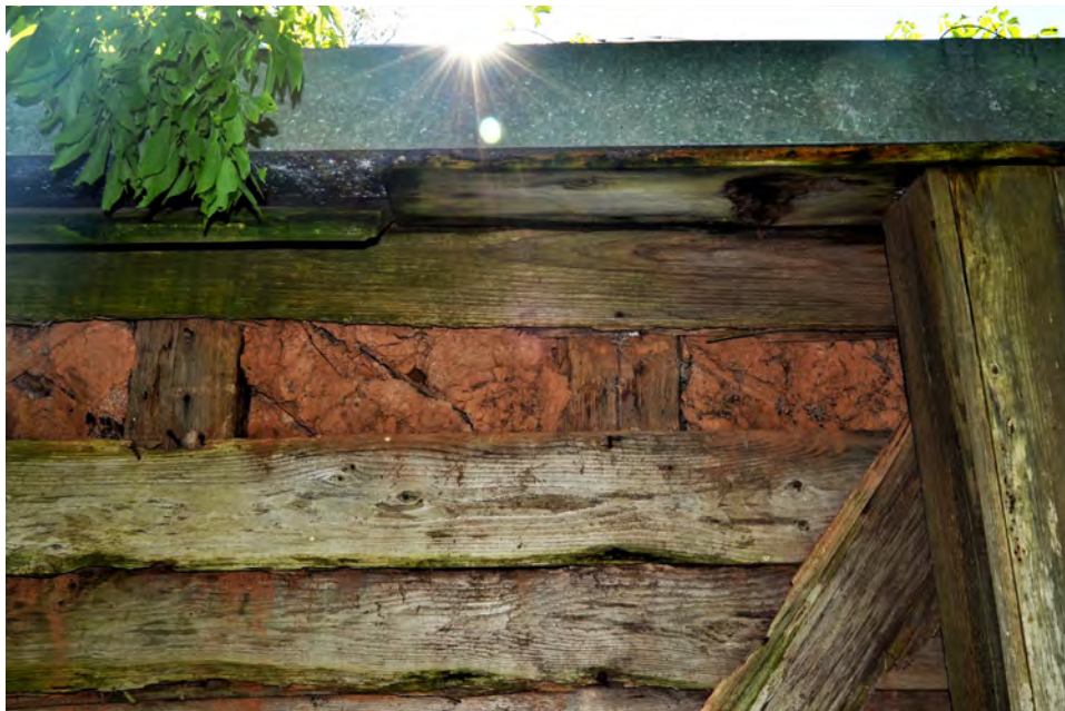
Below: Where the rear gutter has been leaking, several of the vertical posts are completely rotten.
