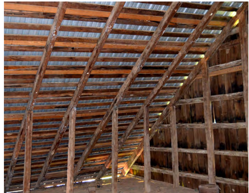
Below: The attic framing lacks sufficient lateral bracing.
