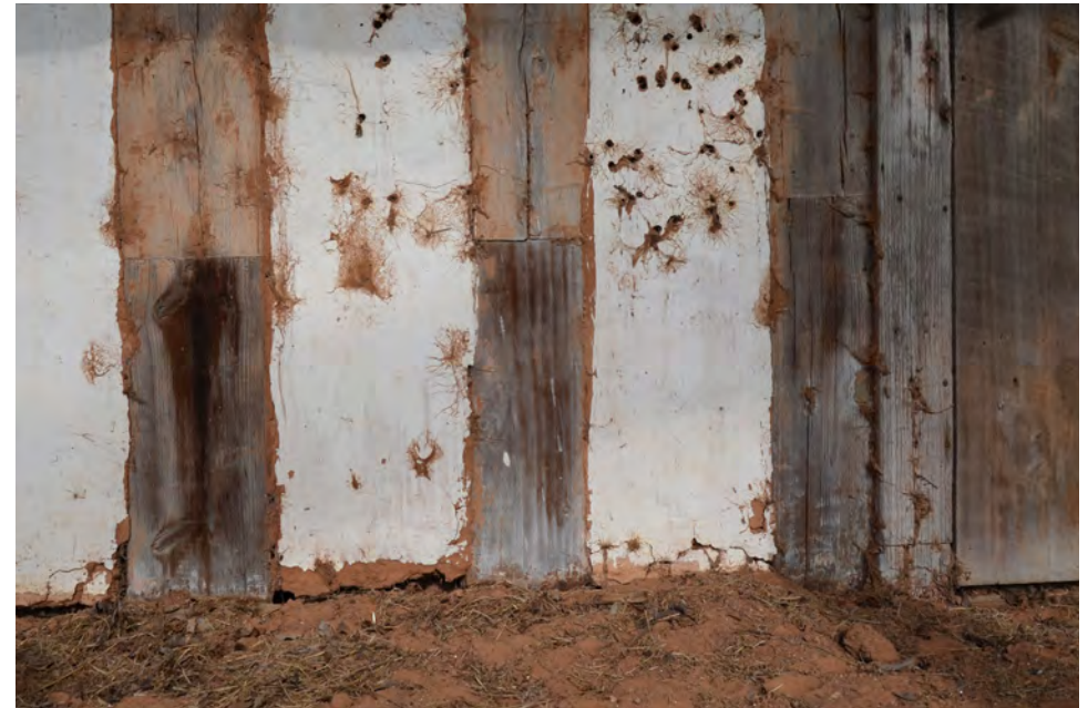
Above: Typical post splices shown at grade. We recommend installing concealed stainless steel side plates at these types of splices (splice plates are diagramed on previous page).
