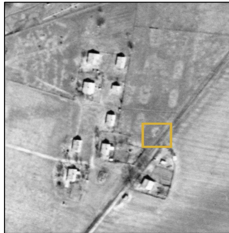
Fig 2.18. A 1955 aerial photograph provides the earliest record showing the cattle dipping vat, highlighted with an orange box. This image reveals the incomplete grid of the eight remaining cabins and the footprints of other cabins. The ruin of Cabin 9 appears as a vegetative blur south of the second row of cabins. Courtesy CARI.
