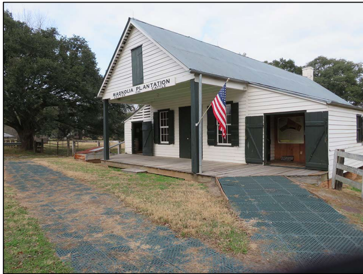
Fig 3.63. Trail mat reinforces the circulation surface with added ramp to facilitate porch access. The contrasting surface detracts from the open, undefined circulation seen in the earlier view. A low stone step is present in the historic location. Missing features include the gas pumps, purple martin birdhouse (relocated to the south), gravel paved frontage and wooden box bench. Heritage Landscapes.
