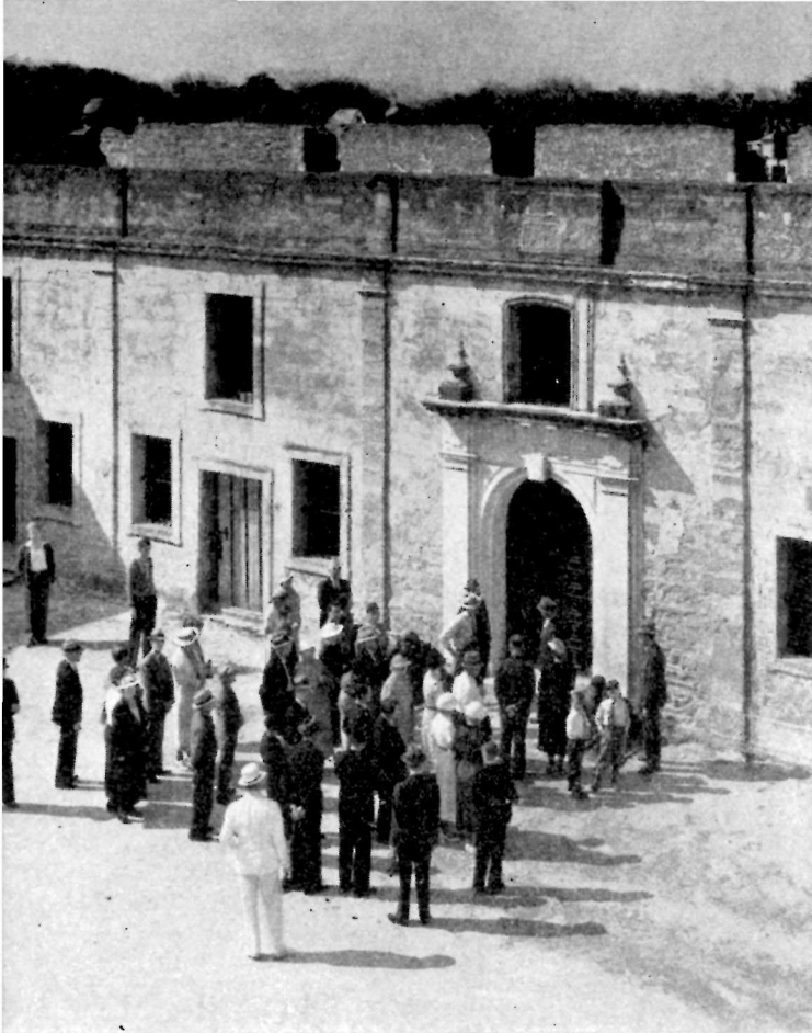
Visitors inspect the rebuilt garrison chapel doorway, originally designed by a Spanish engineer in 1785. Almost all the rooms open into the courtyard, which is about 100 feet square. Rooms were used variously as quarters, storerooms, and prisons. In many of the rooms the English built a second floor.
