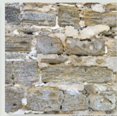
Cut stone walls © NPS / BETSY EHREICH
