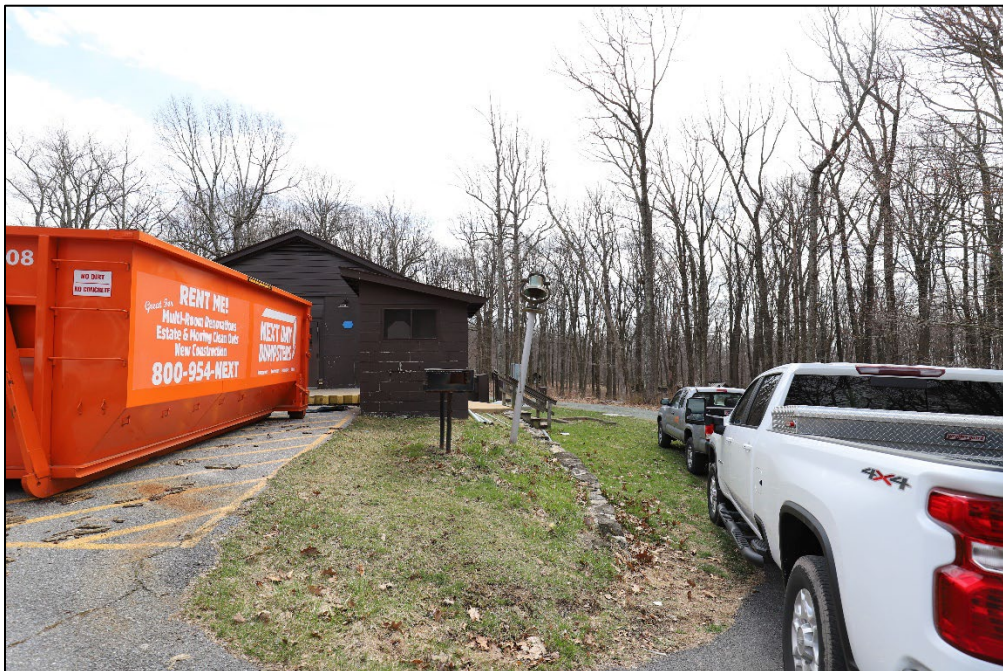
Fig 62: Dinner bell, large grill, mop house, retaining wall, and loading dock viewed to the east adjacent to the recreation hall. (NCR 2023)
