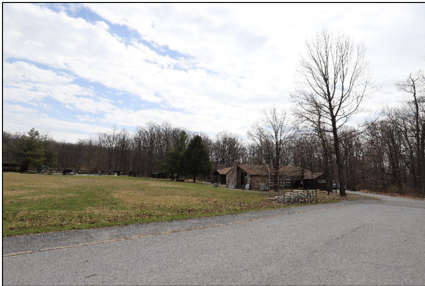
Fig 47: Overall of Camp Greentop, viewed to the southeast towards the playing field and dining hall and kitchen and recreation hall facility.
