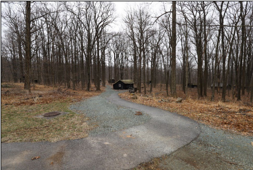
Fig 29: Asphalt paved pedestrian walkway paved over main gravel loop road. (NCR 2023)
