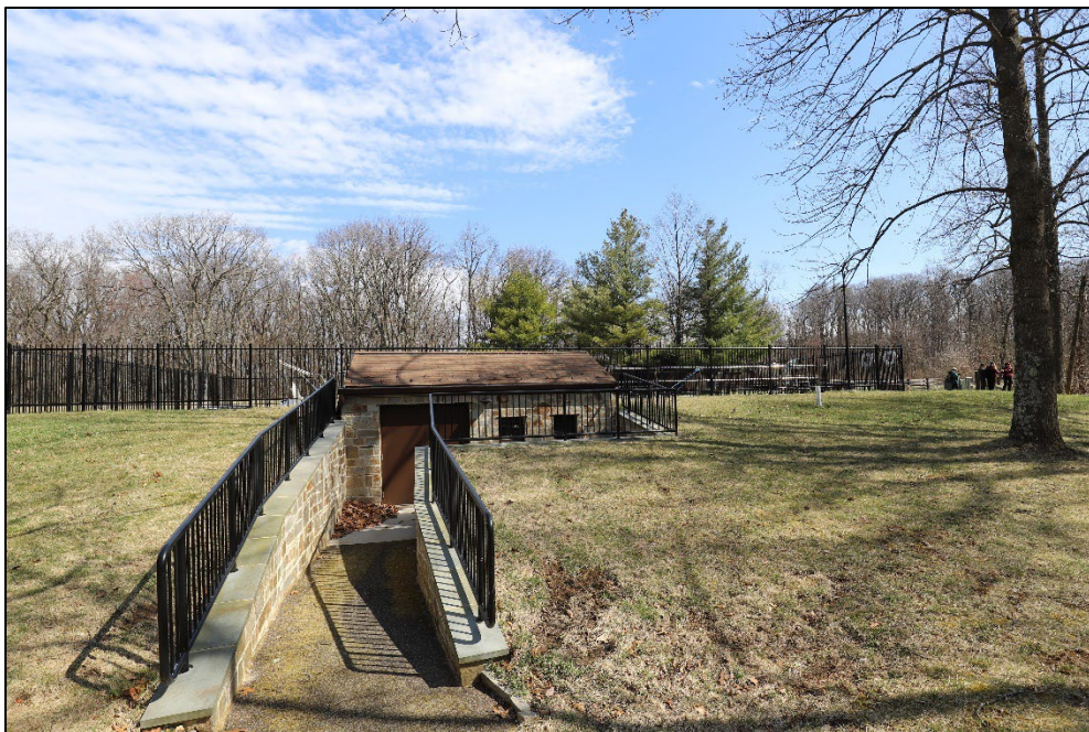
Fig 52: Pump house on the south side of the swimming pool constructed during the 2018 pool replacement project. (NCR 2023)
