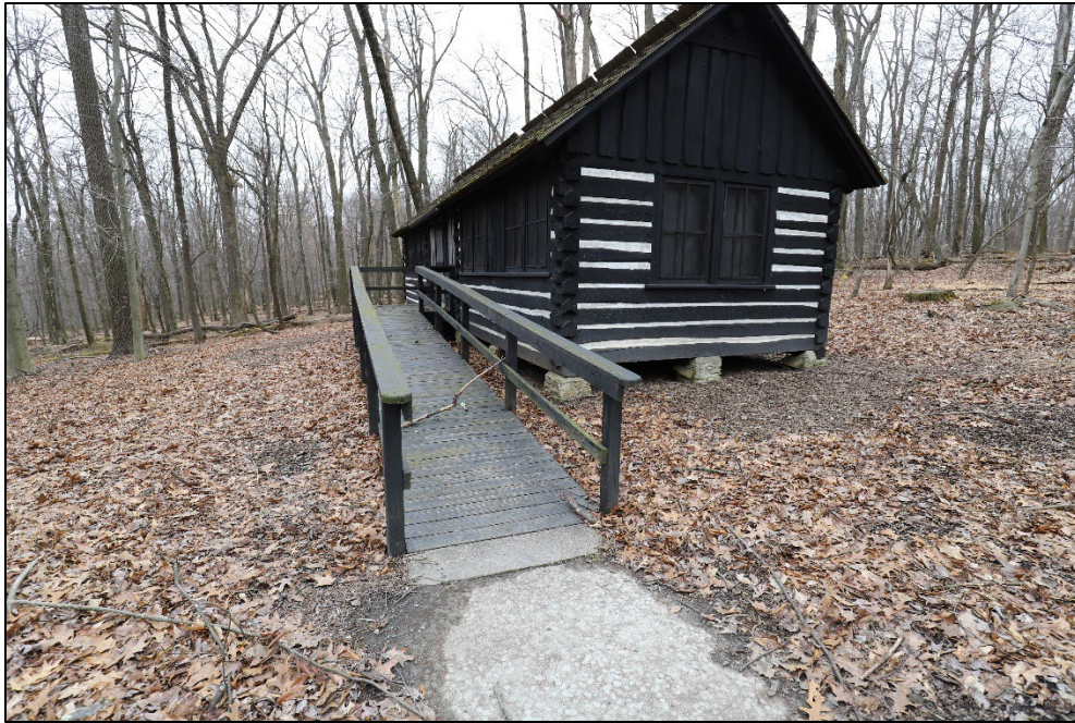
Fig 41: Wooden accessible ramps that provide access to cabin camps. (NCR 2023)
