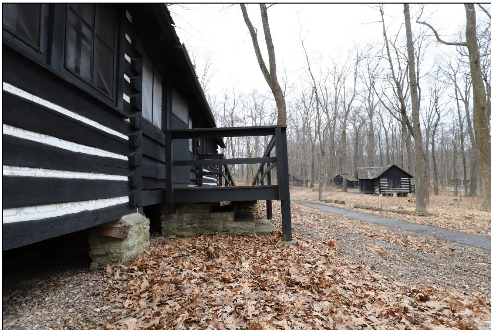
Fig 40: Remnant stone steps underneath wooden accessible ramp of cabin. (NCR 2023)
