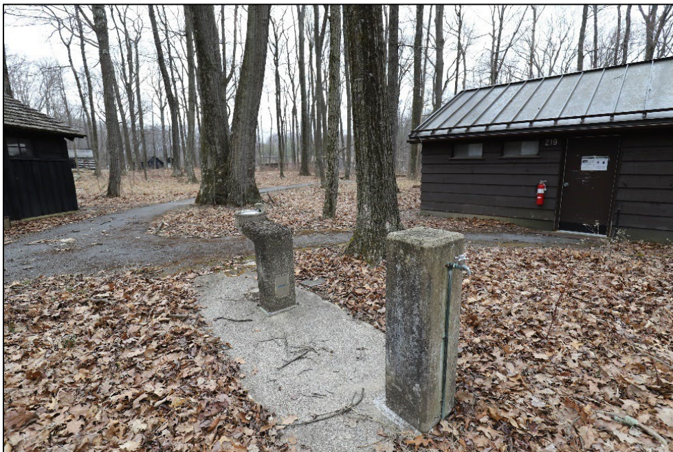
Fig 64: Representative photo of one of five contemporary drinking fountains. (NCR 2023)
