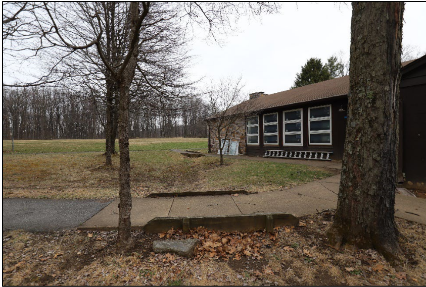
Fig 30: Concrete walkways outside dining hall. (NCR 2023)
