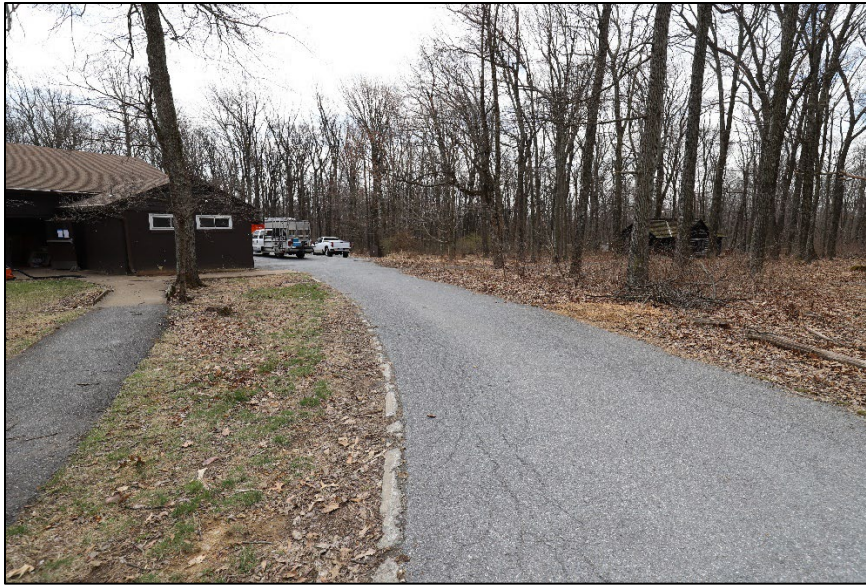
Fig 32: Main gravel loop road (partially paved with asphalt) leading to loading dock area. (NCR 2023)
