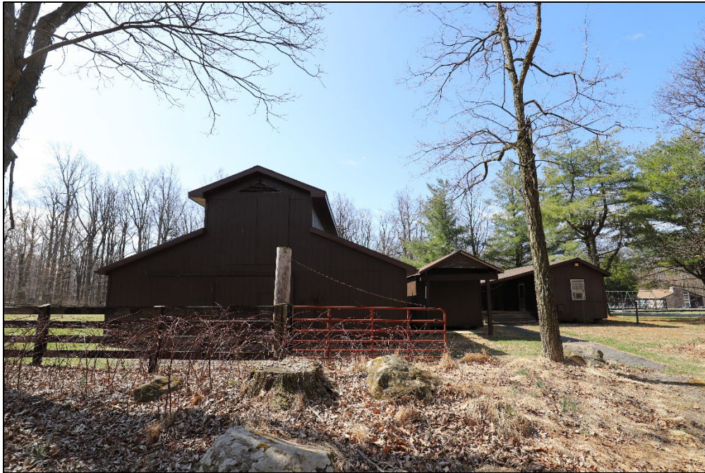
Fig 43: Noncontributing stable and tack room (left) and stable office. (NCR 2023)
