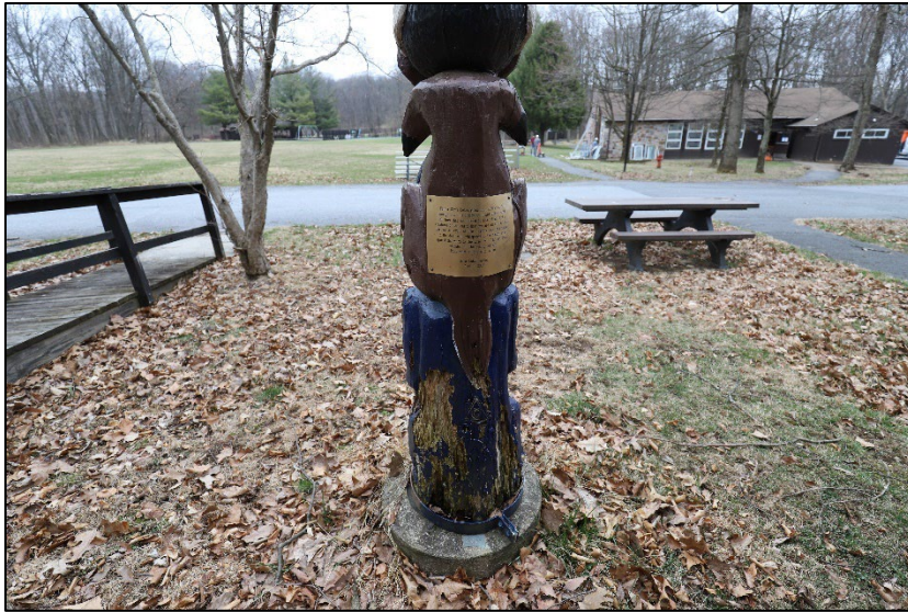
Fig 59: Deterioration at the base of the totem pole. (NCR 2023)
