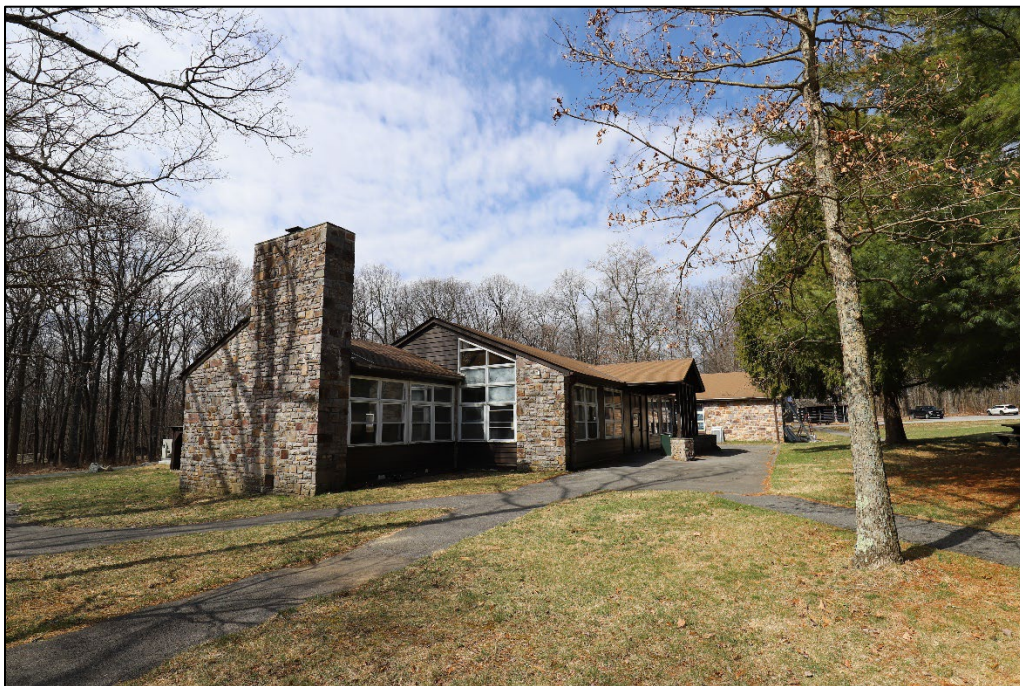
Fig 38: Contributing dining hall and kitchen and recreation hall. (NCR 2023)
