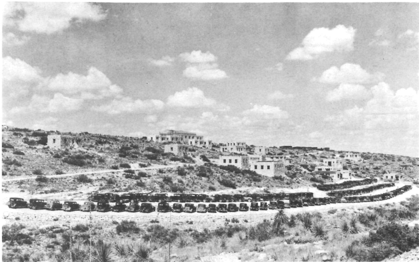
PARKING TERRACES AT CAVERNS ENTRANCE
