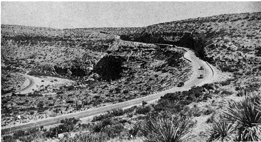
WALNUT CANYON HIGHWAY
