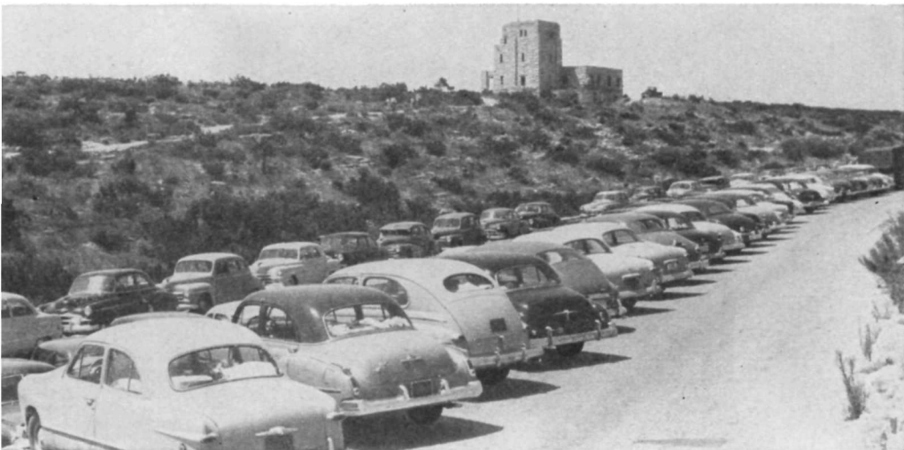
LOWER PARKING TERRACES AND ELEVATOR BUILDING
