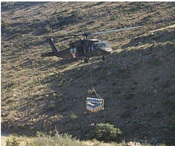
A Military Helicopter Ferries Culvert Pieces To The Lechuguilla Cave Entrance. (NPS Photo by Fred MacVaugh)
