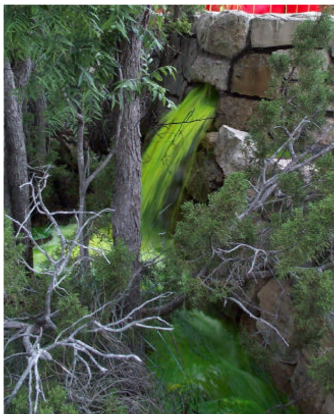
Water with fluorescein dye runs off Bat Cave parking lot. (NPS Photo by Paul Burger)
