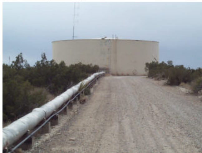
NOW YOU SEE IT! The 500,000-Gallon Water Tank on March 17, 2001. (NPS Photo by Dale Pate)
