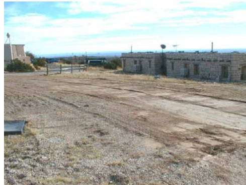
GONE! Open space where the playground use to be. (NPS Photo by Renée West)
