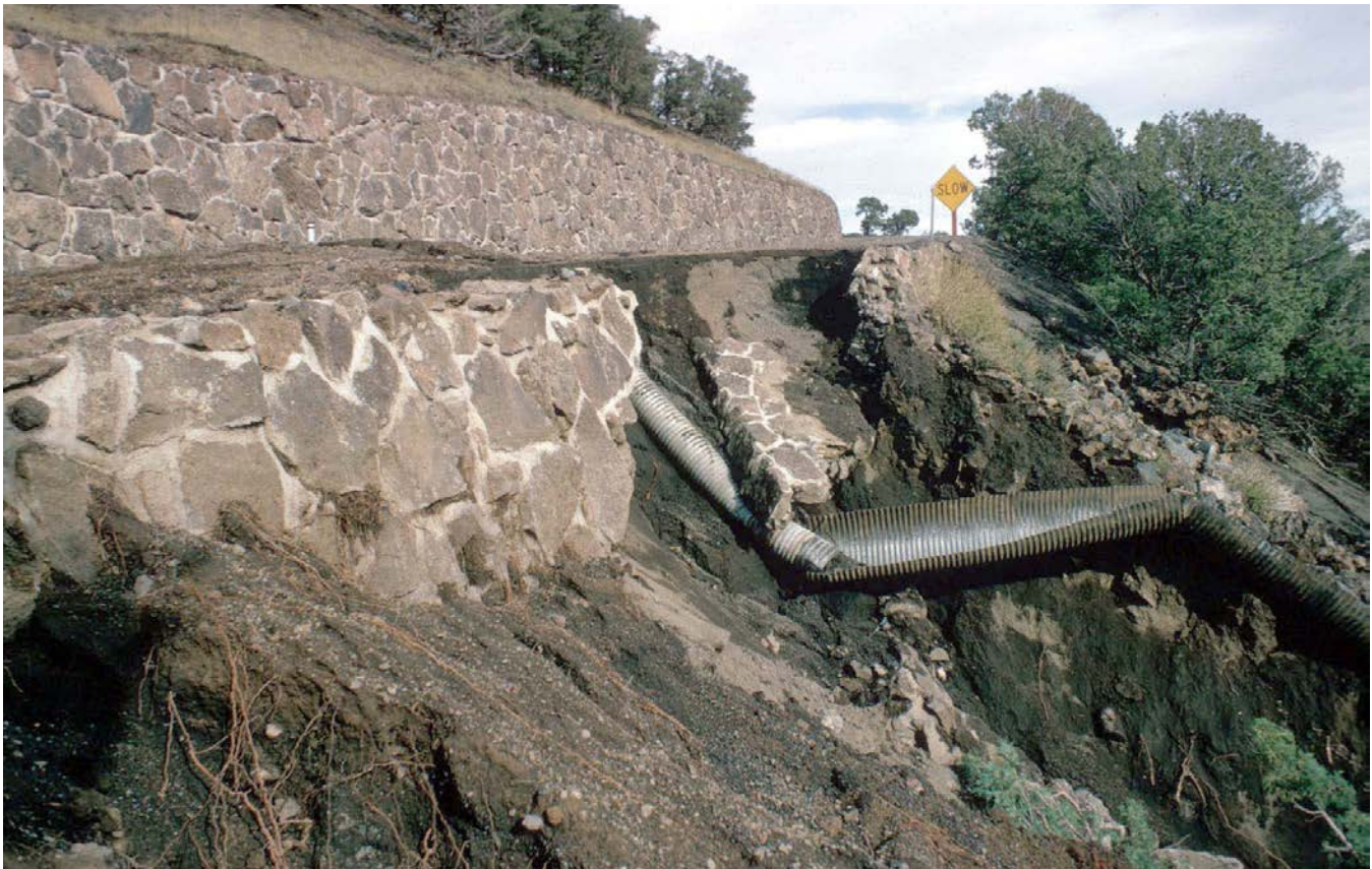
Figure 28. Photograph of storm-related damage along Volcano Road. Erosion on Capulin Volcano is primarily associated with Volcano Road. Culverts provide narrow paths for storm-water runoff, creating erosion channels and gullies down the sides of the mountain. National Park Service photograph (date unknown).
