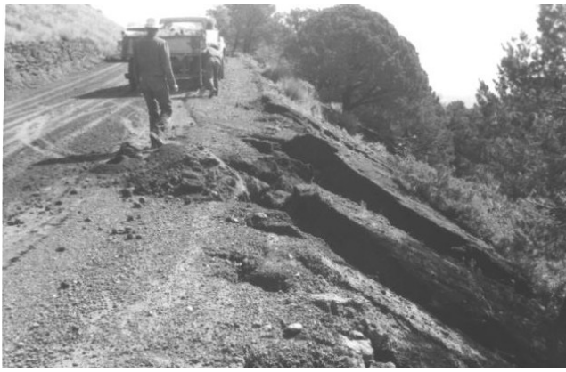
Figure 30. Photograph of erosion along Volcano Road. In spring 1967 Volcano Road was closed while monument personnel assessed damages and made repairs. In 2012, a Federal Highways Administration project remediated some areas of severe erosion along the road. National Park Service photograph from Bennetts et al. (2012, figure 4.5.1-7).
