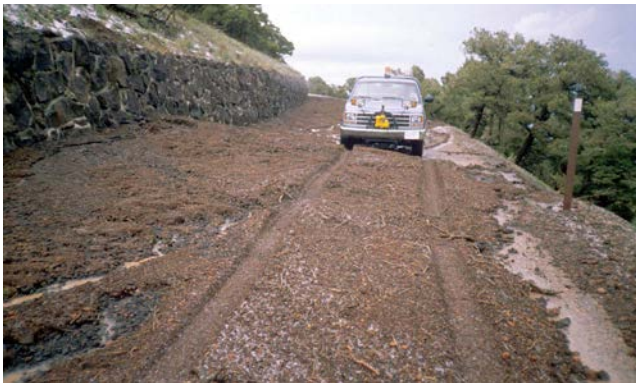
Figure 32. Photograph of a debris flow on Volcano Road. Slope movements are a common type of geologic hazard—a natural or human-caused condition that may impact park resources, infrastructure, or visitor safety. Debris flows have impacted Volcano Road, causing road closures and trapping vehicles above an affected road section. National Park Service photograph (date unknown).
