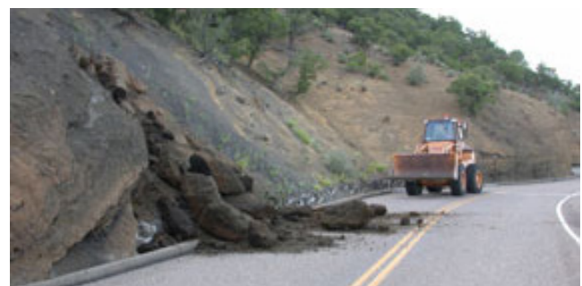
Figure 31. Photograph of a cinder slide on Volcano Road. Slope movements are ongoing at Capulin Volcano National Monument; the slide shown here took place in 2004. Cinder slides are a particular concern along Volcano Road. Keeping the road clear of cinders is a continuous maintenance activity. National Park Service photograph available at http://www.nps.gov/cavo/naturescience/environmentalfactors.htm (accessed 19 November 2014).
