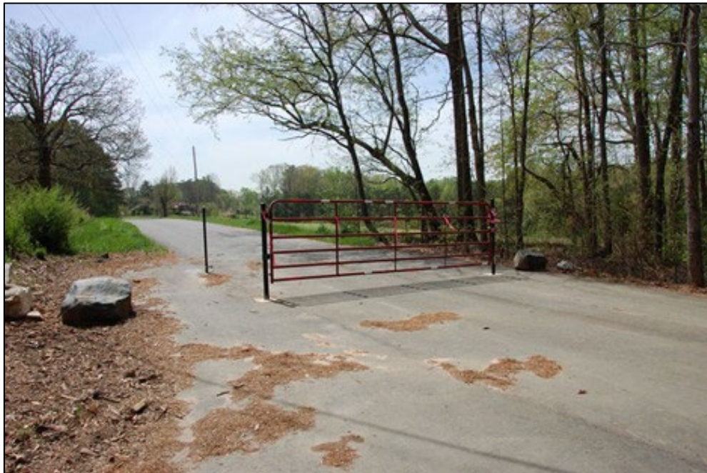
Fig 44. New Cobb County gate across Hyde Road, 2010.
