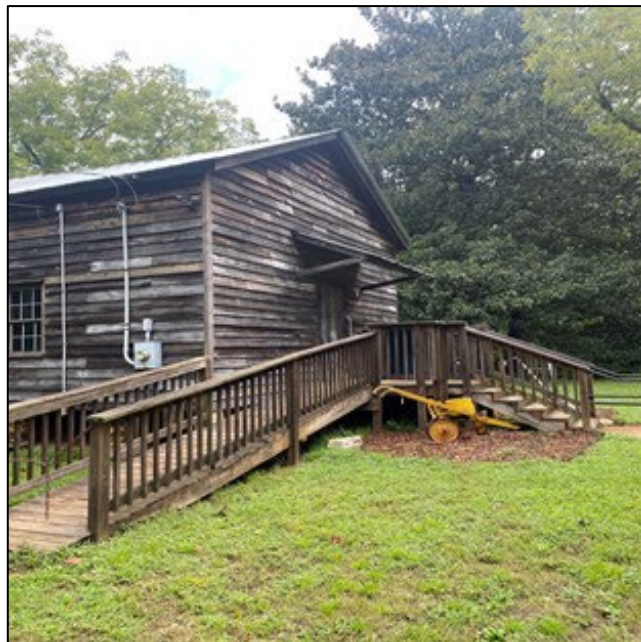
Fig 30. Rear ell of Power-Hyde House, showing ramp, 2022.
