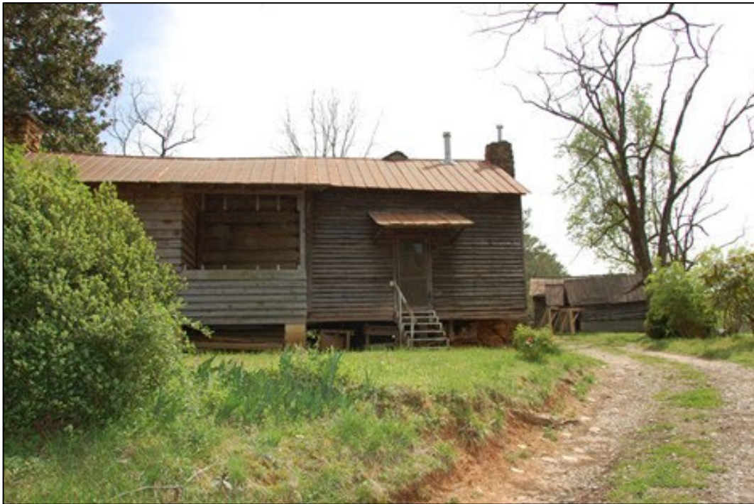
Fig 28. North elevation of the Power-Hyde House.
