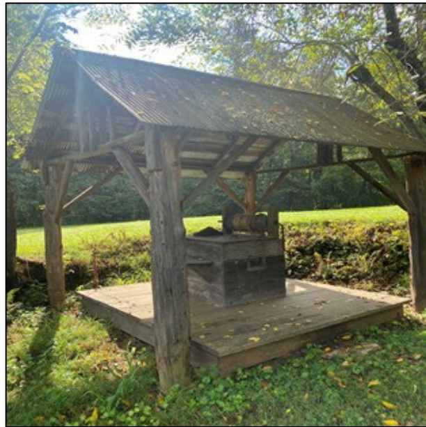
Fig 23. Well and well house, 2022.
