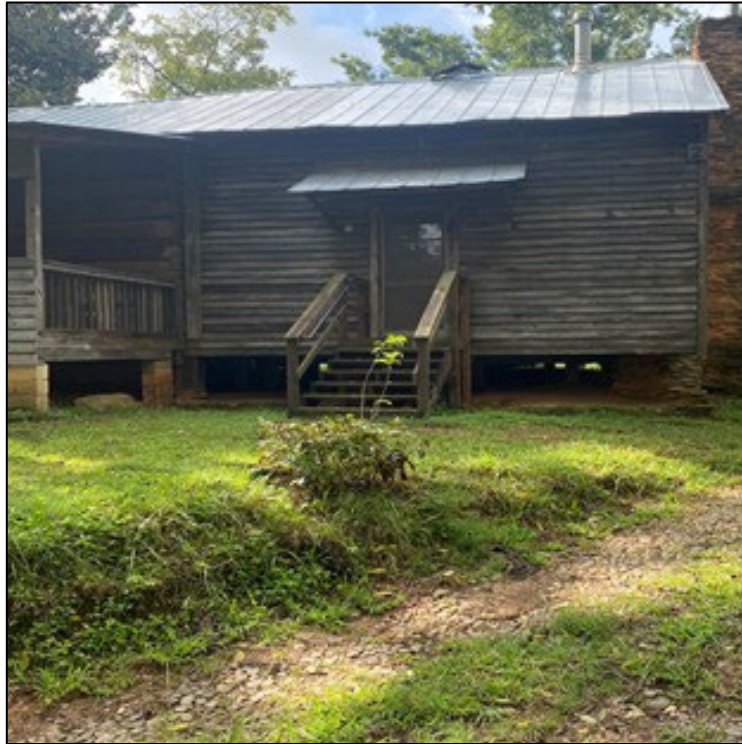
Fig 29. North elevation of the Power-Hyde House, 2022.
