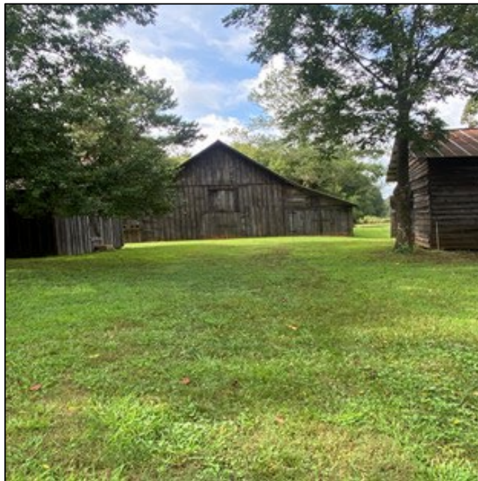
Fig 64. Work yard behind house, 2022.
