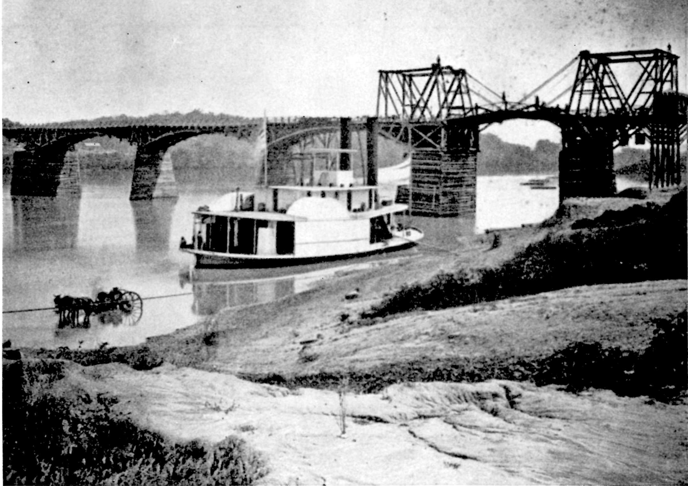
The Federal Army built this trestle bridge across the Tennessee River during the Chattanooga campaign. (Signal Corps, U. S. Army)
