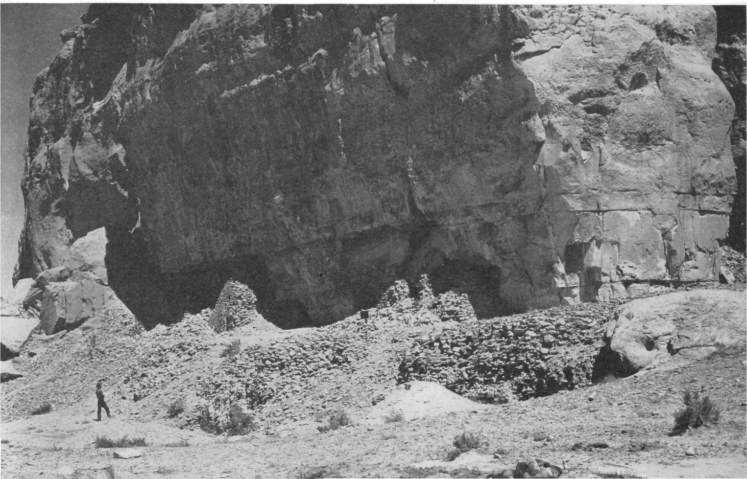
View of Threatening Rock, prior to its fall, showing masonry constructed at its base by the Indians in an attempt to prevent its collapse on Pueblo Bonito.
