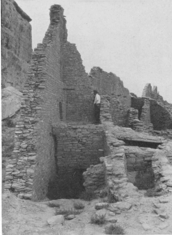
Cross section view of a portion of Pueblo Bonito ruins showing types of masonry and exposed floor beams.
