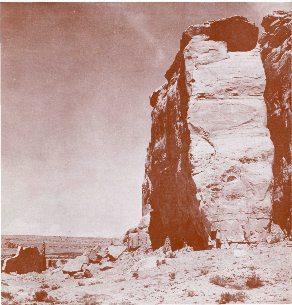
Threatening Rock before it fell on January 22, 1941.
