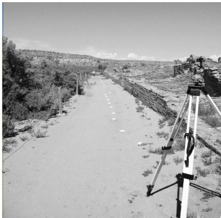
Figure 49. Theodolite position at Pueblo Bonito's south wall, west section Among all the features identified as aligned to the cardinal directions in surveyed Chacoan architecture, this wall section is the most accurate and precise.
