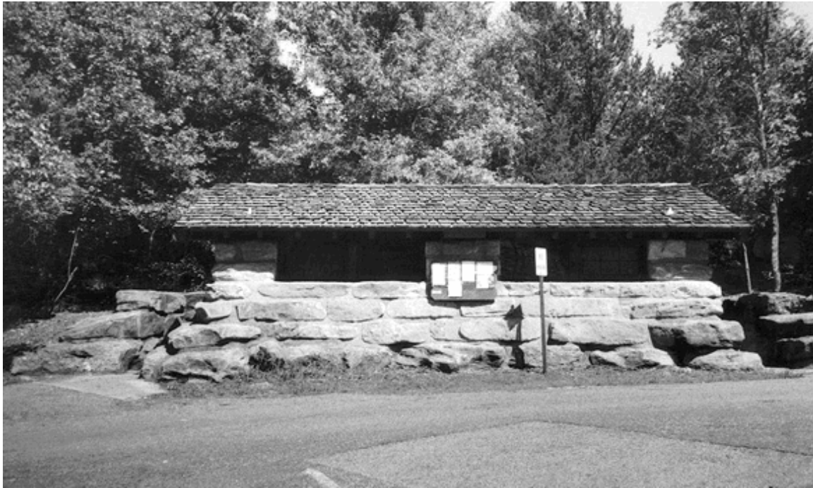
Central Campground comfort station, circa 1999. (CNRA archives, LCS photograph)
