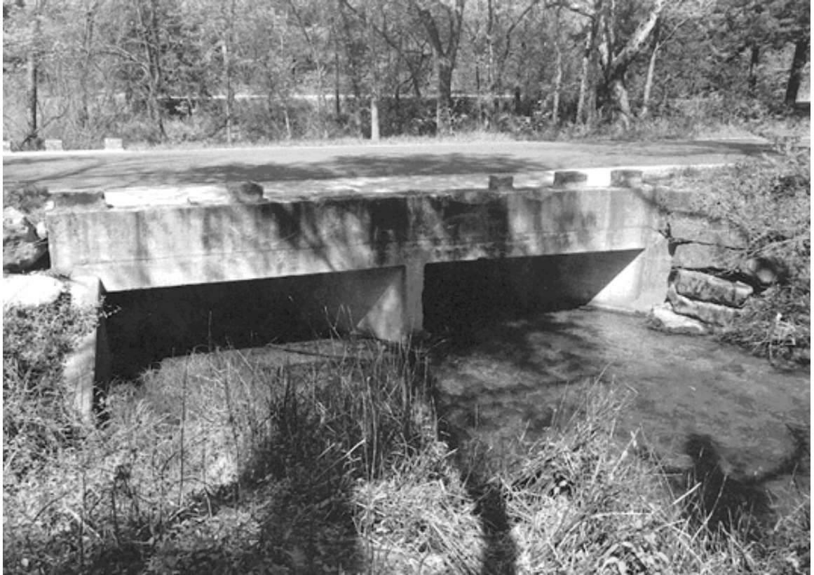
Panther Falls bridge culvert, circa 1995. (CNRA archives, LCS photograph)
