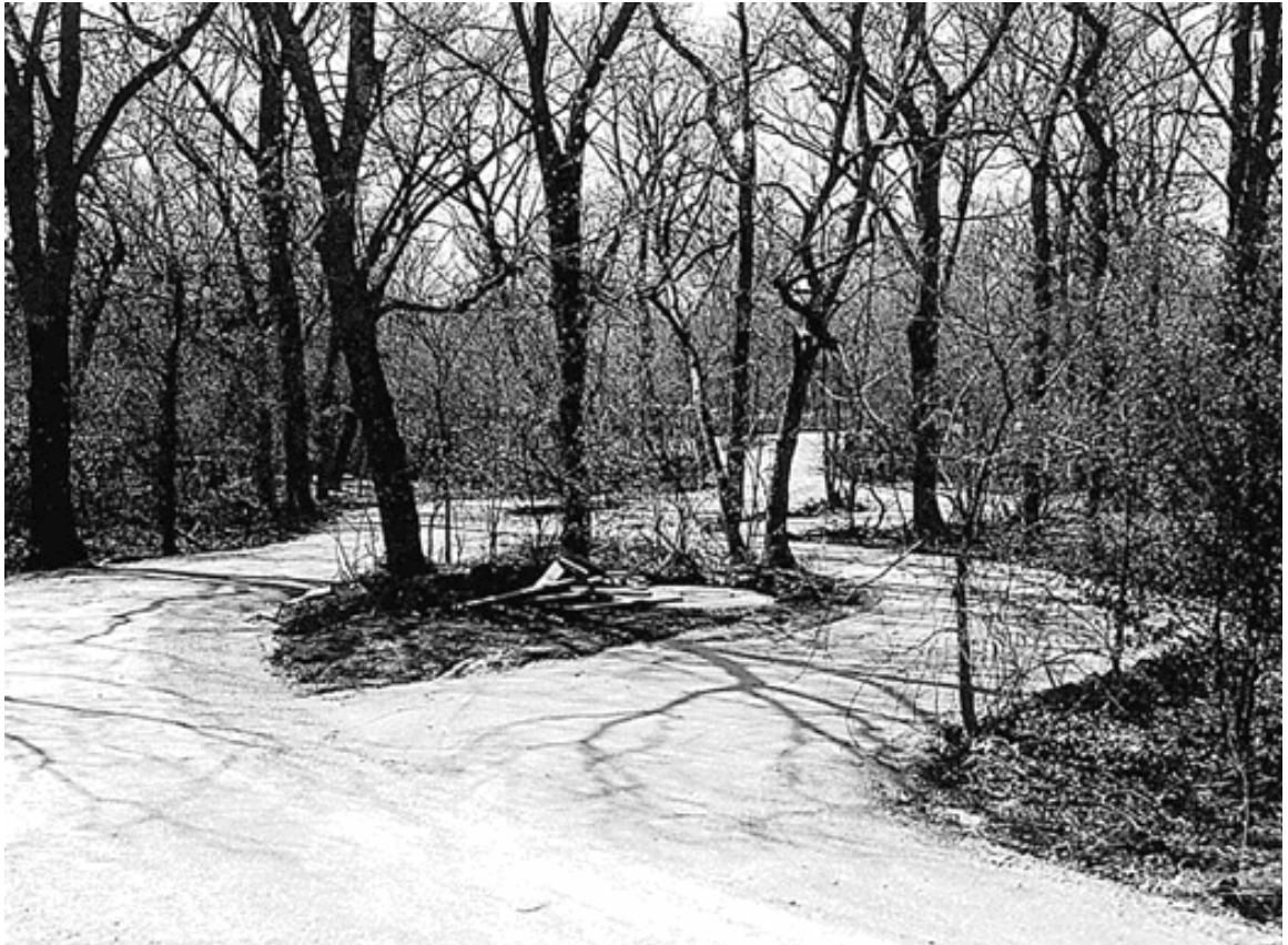
Extension of Rock Creek loop road system, showing alternating campsite drive-through access pattern, 1966. (CNRA archives, photograph RC-511)
