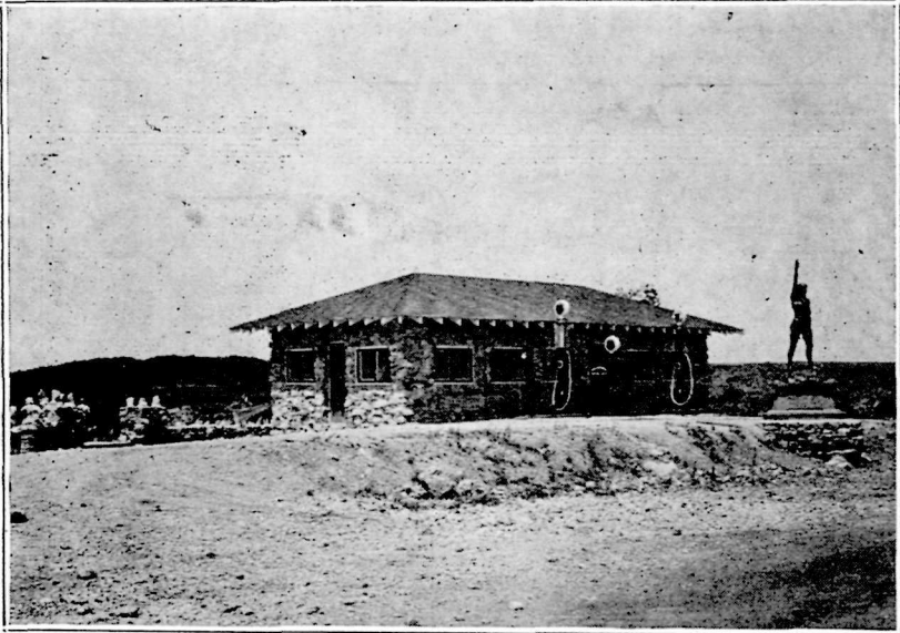
STATION AT TURNER FALLS
