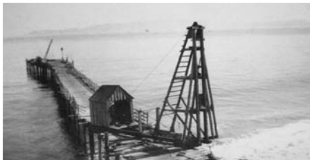
The pier with pile driver in operation.
