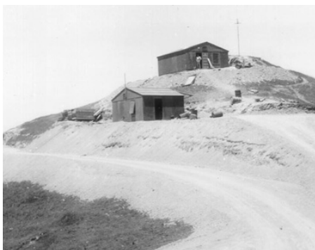
Radar building on Soledad Peak, 1944.
