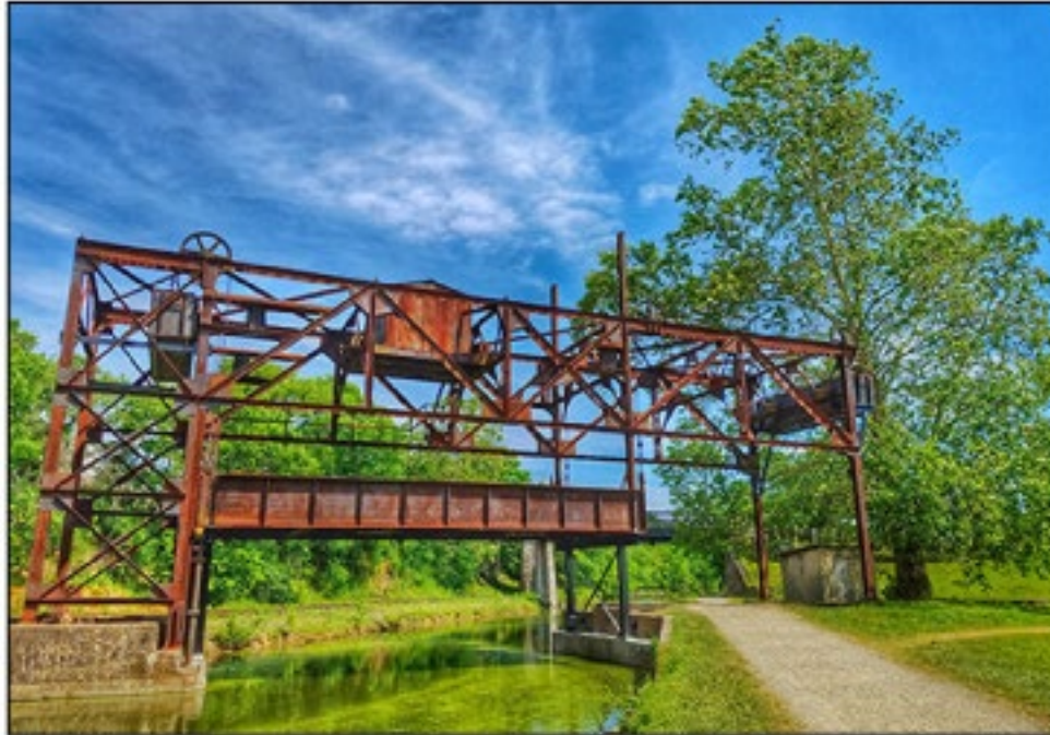
FIGURE 4.7: Western Maryland Railroad Lift Bridge at Williamsport
