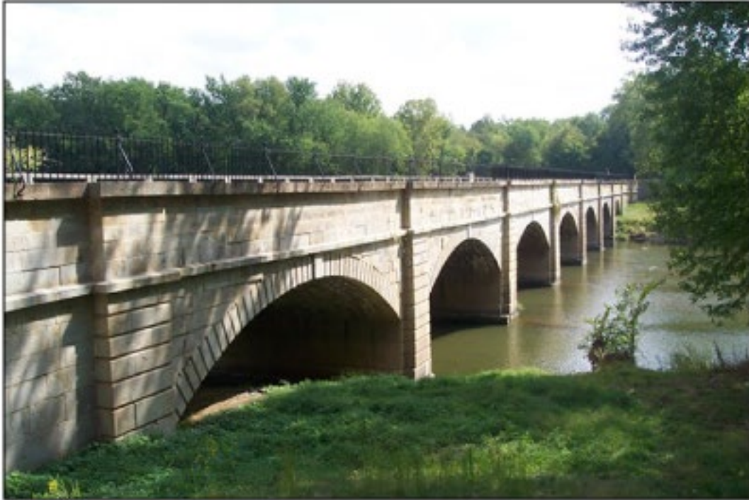
FIGURE 4.5: Restored Monocacy Aqueduct (NPS)
