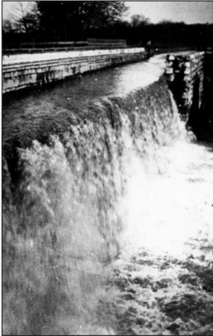
FIGURE 2.6: View of the Conococheague Aqueduct Breach, ca. 1920 (NPS)
