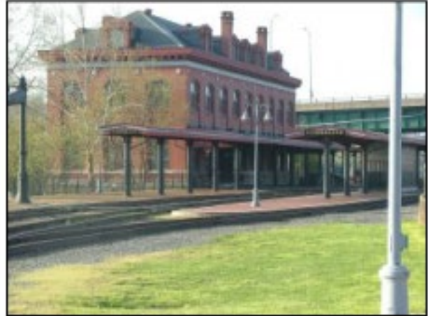
FIGURE 2.11: View of Cumberland Visitor Center and Museum, Cumberland, Maryland (Tina Yoder, 2021)
