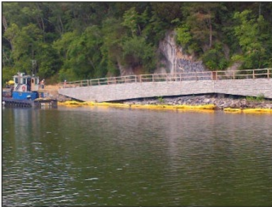
FIGURE 2.5: View of Restored Big Slackwater Towpath, 2012 (NPS)
