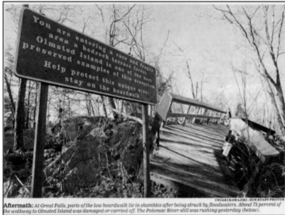
FIGURE 4.3: Newspaper Image Showing Damage to Boardwalk near Great Falls ( Baltimore Sun , January 26, 1996, 21)
