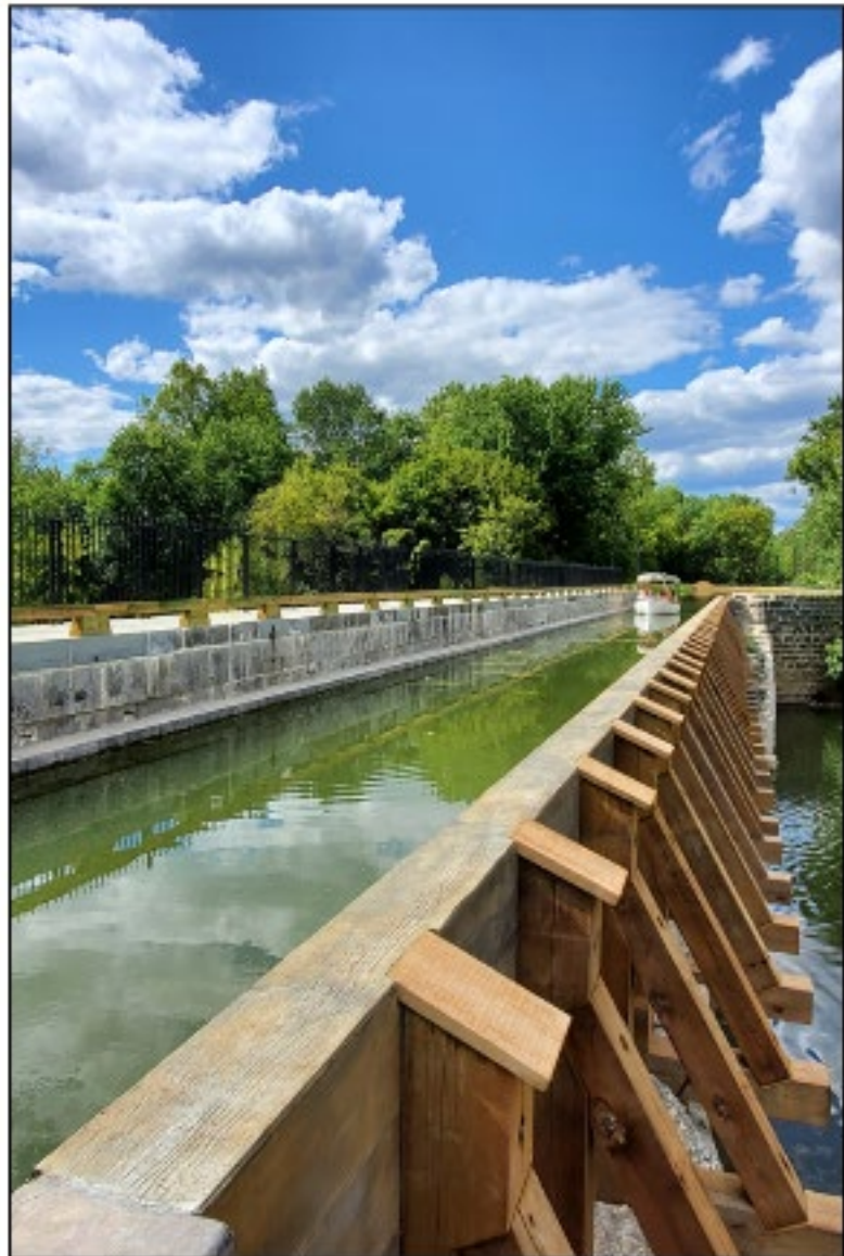
FIGURE 2.7: View of the Restored Conococheague Aqueduct (No. 5), 2019 (Tim Ware, NPS)
