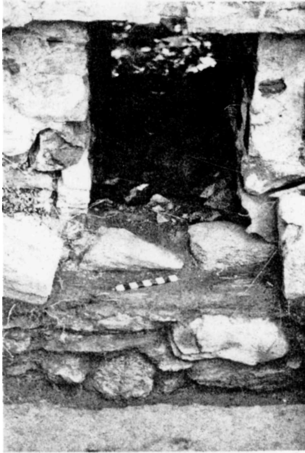
PLATE 6 VIEW OF FEATURE #4 LOOKING EAST THROUGH THE DRAIN HOLE OF THE DRY DOCK
