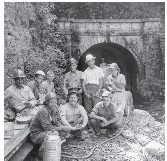
The National Park Service conducted repairs to the tunnel in 1956, 1979, and 2007. Above, craftsmen repairing the tunnel take a lunch break.
