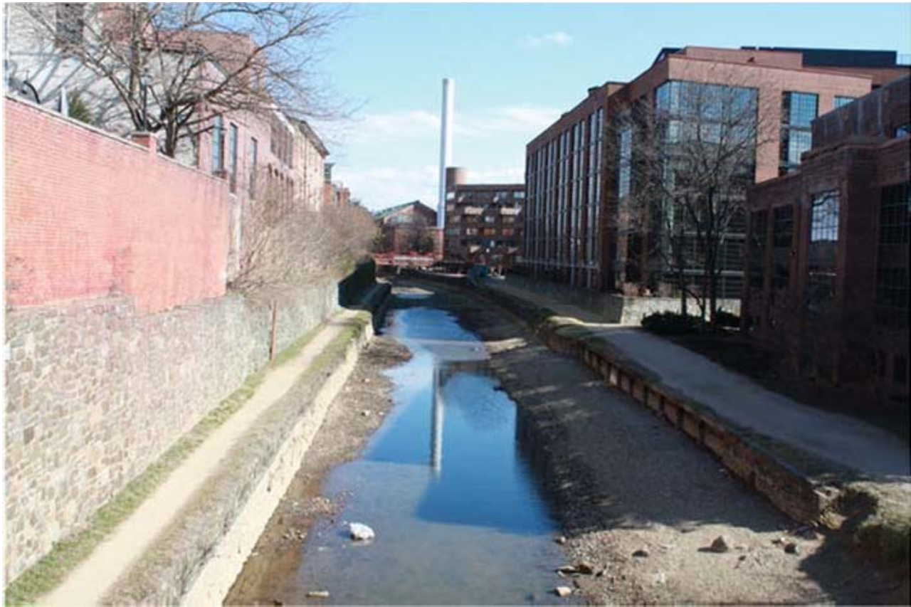
This view west to Potomac Street illustrates how construction has encroached on the canal on both the river and berm side of the canal between 33rd and 34th Street. (NCR CLP 2017).
