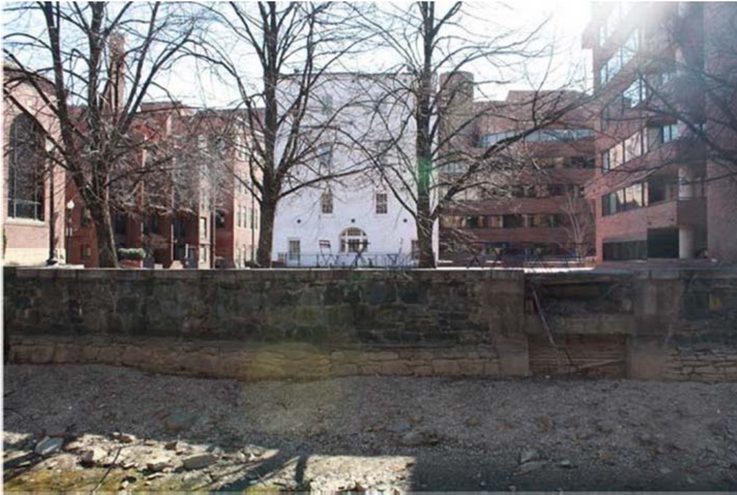
The Fish Market Square, designed by Peter Vercelli. This photograph also captures the Dual Water Intake-Ruins of the Wilkins Rogers Milling Co., which supplied the former mill to the south with surplus canal water from 1839 to 1960. (NCR CLP 2017).
