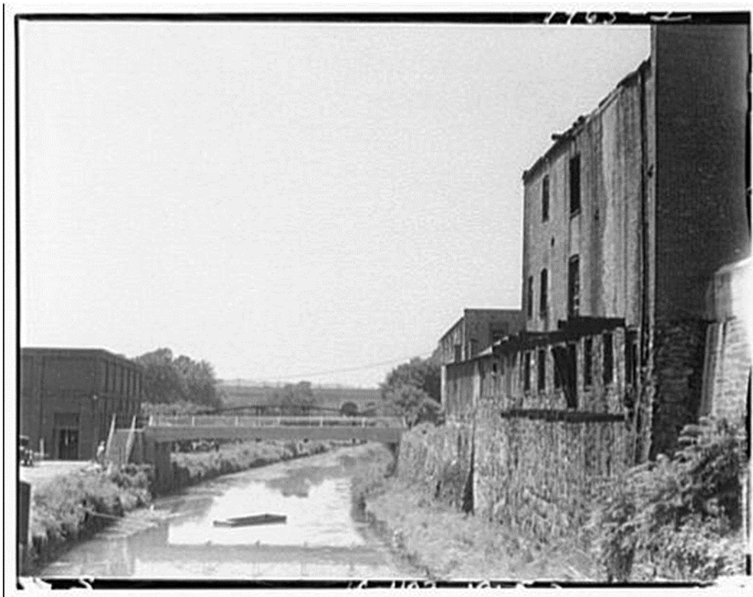
The Potomac Street Bridge circa. 1920-1950. "Chesapeake and Ohio Canal (C&O Canal) Canal in Georgetown. C&O Canal View I." Theodor Horydczak, ca.1920-1950. From the Library of Congress ( https://www.loc.gov/item/thc1995004371/PP/ , accessed 2017).
