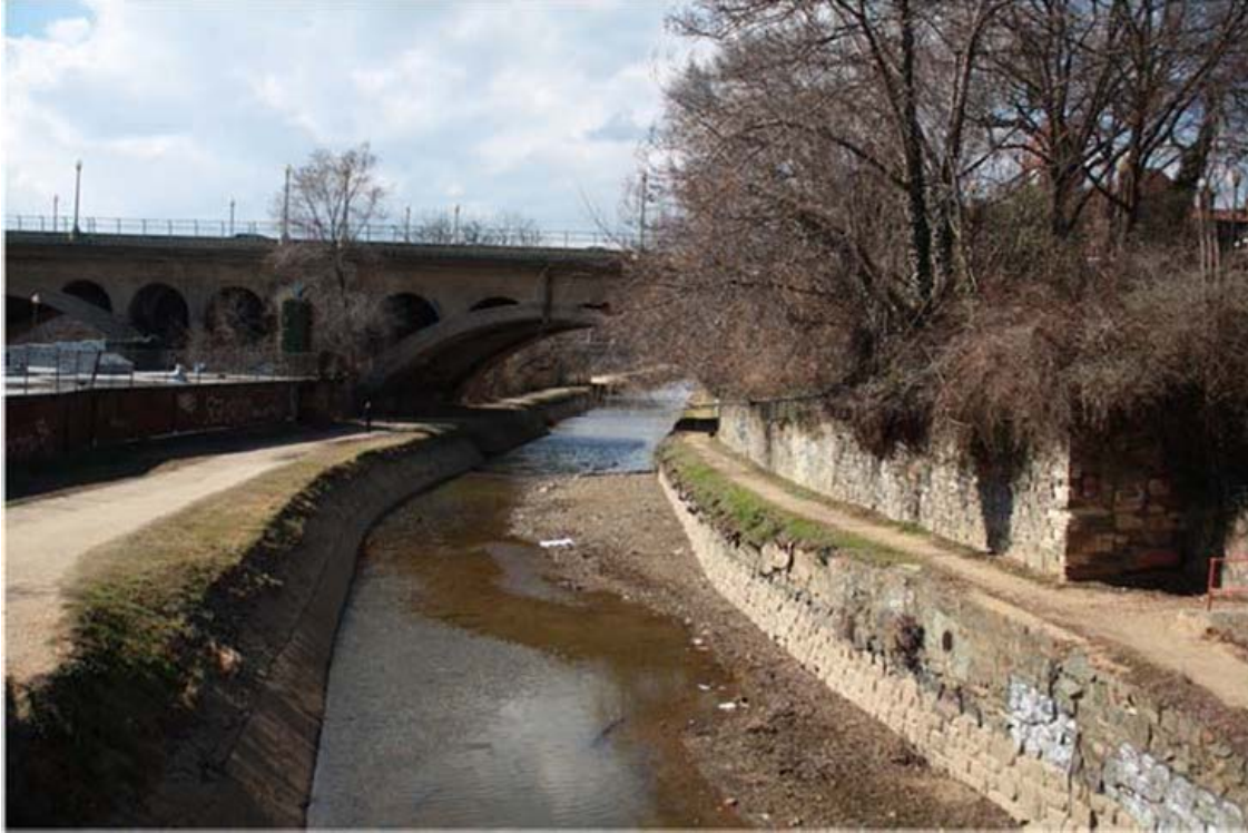
The views along the canal west to the Key Bridge. (NCR CLP 2017).
