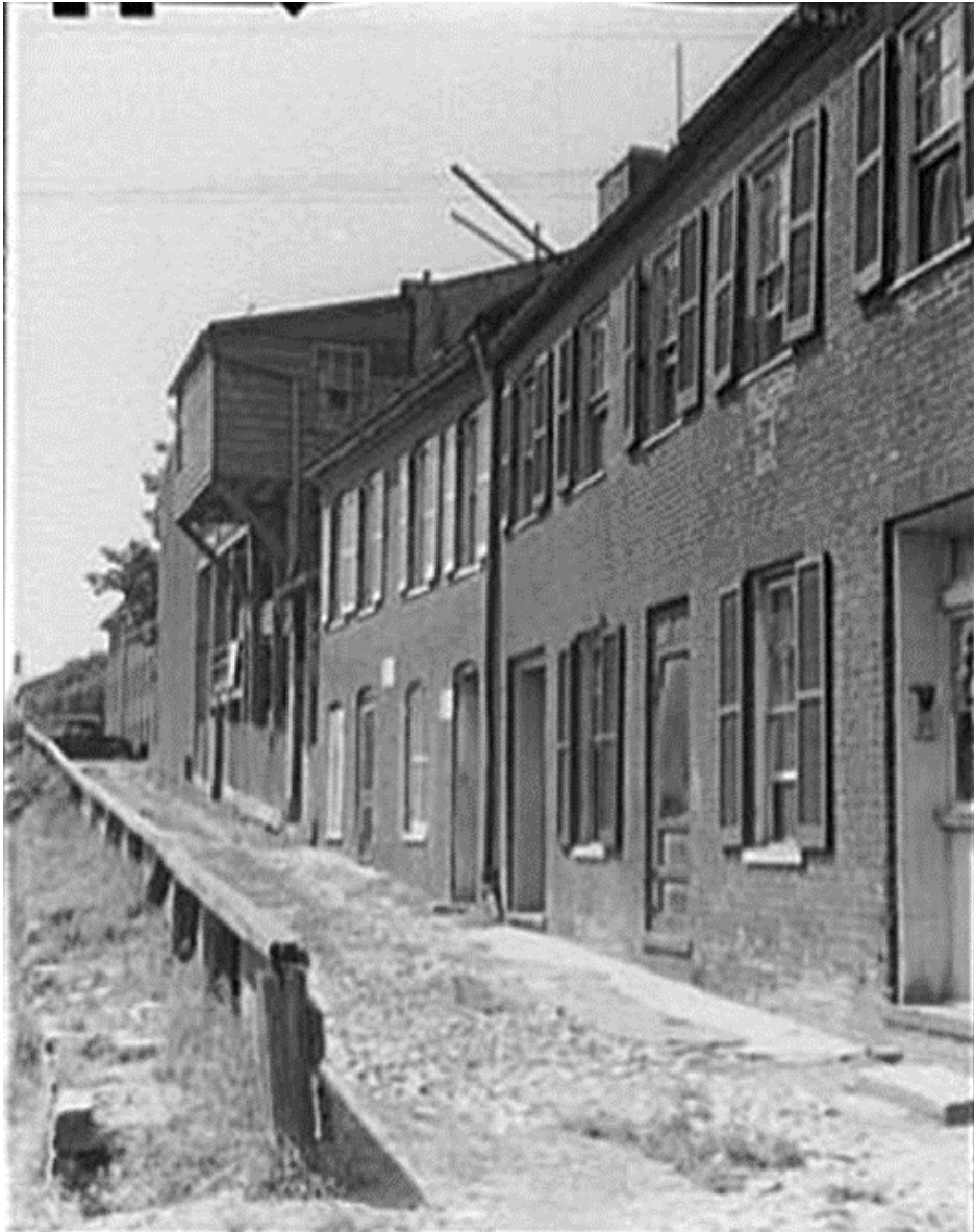
In this photograph, a possible cobble stone path is present on the berm side of Chesapeake and Ohio Canal of Lock 4 "(C&O Canal) Canal in Georgetown. Path along C&O Canal." Theodor Horydczak, ca. 1920-1950. From the Library of Congress ( https://www.loc.gov
