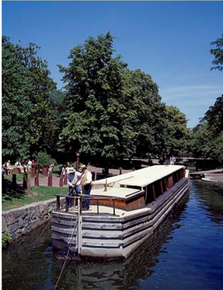
Photograph of Lock No. 3 looking west. "Tourist barge on the old C&O Canal in the Georgetown section of Washington, D.C." Carol M. Highsmith, 1980. From the Library of Congress ( https://www.loc.gov/item/2011632165/ , accessed 2017.)
