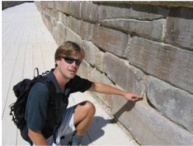
Figure 1.14 Corner weathering at the Monocacy Aqueduct of the C&O Canal. These blocks of quartzite from nearby Sugarloaf Mountain (not the “white granite” described in the Canal Company proclamation posted at the parking area nearby) show preferential weathering at their corners. Why?
