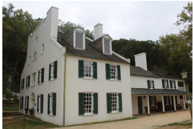
Figure 159: North Wing Viewed from Northwest (Silman 2019)
