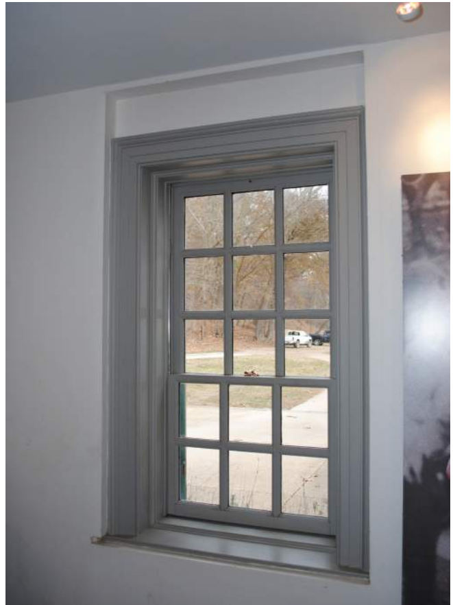
Figure 130: North Wing First Floor, East Window in South Wall (BBB 2019)
