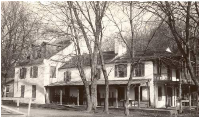
Figure 40: South and West Elevation, Looking Northeast, 1939. (CHOH NHP)
