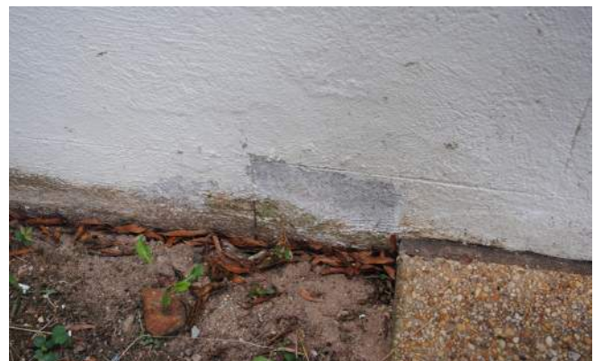
Figure 111: Stucco Scratch Coat at Foundation (BBB 2019)
