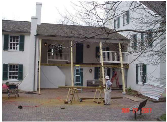
Figure 95: Reconstructing East Porch, March 27, 2007. (NPS)
