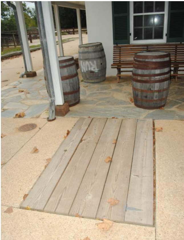
Figure 123: Closed Cellar Door South of South Elevation, Looking North (BBB 2019)
