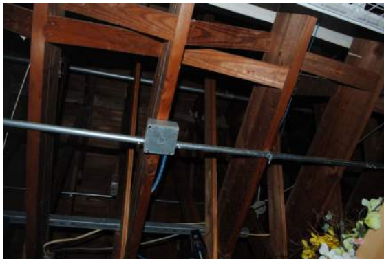
Figure 194: Roof Framing, North Wing (BBB 2019)
