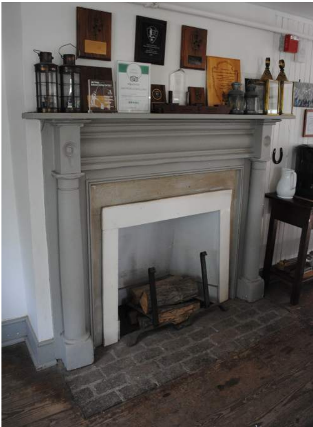
Figure 151: South Wing, Second Floor Fireplace (BBB 2019)
