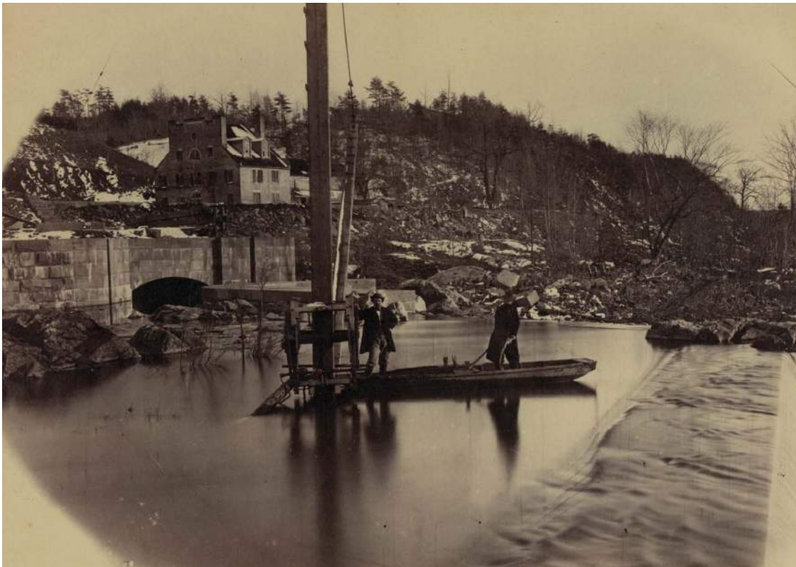
Figure 17: Washington Water Works With Tavern Beyond, 1861-1865. (Library of Congress)
