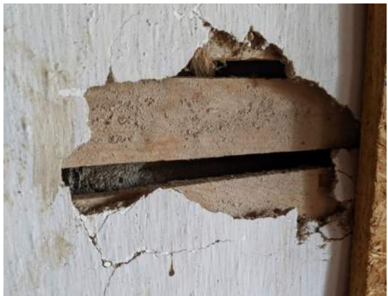
Figure 215: Historic Plaster Applied to Wood Lath on Third Floor (BBB 2019)
