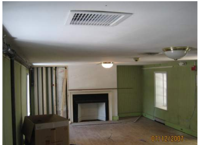
Figure 107: Center Section Second Floor Under Construction, July 12, 2007. (NPS)
