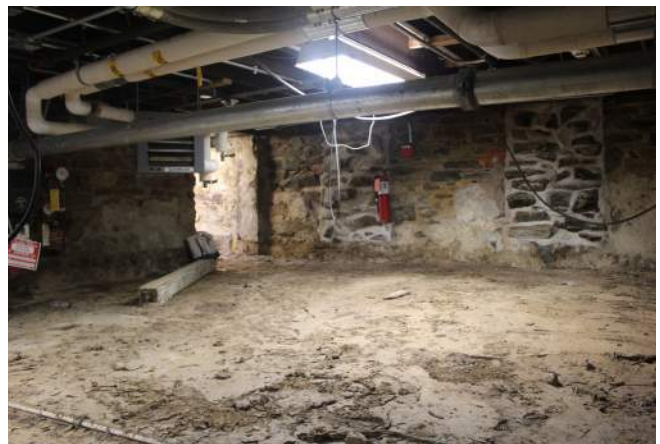
Figure 164: South Wing Cellar Looking Southwest (Silman 2019)
