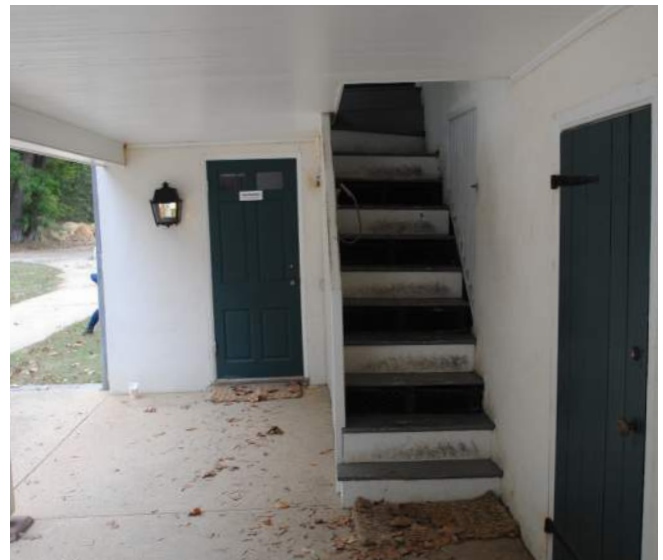
Figure 114: East Elevation Porch at First Story, Looking South (BBB 2019)
