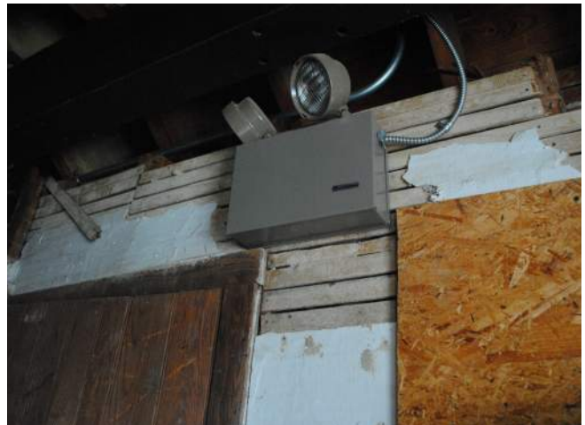
Figure 157: North Wing Attic, Partition Looking East (BBB 2019)
