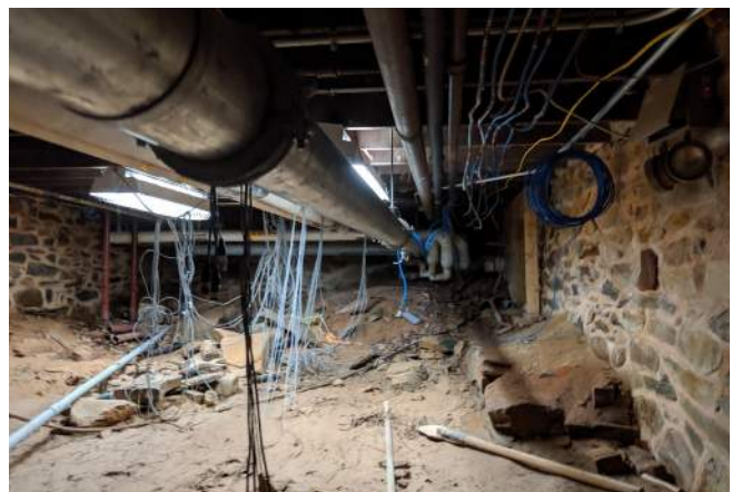
Figure 127: Center Section Cellar Looking Northeast. (BBB 2019)
