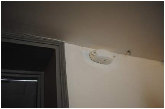
Figure 216: Replacement Plaster Applied to Metal Lath on Center Section, First Floor (BBB 2019)
