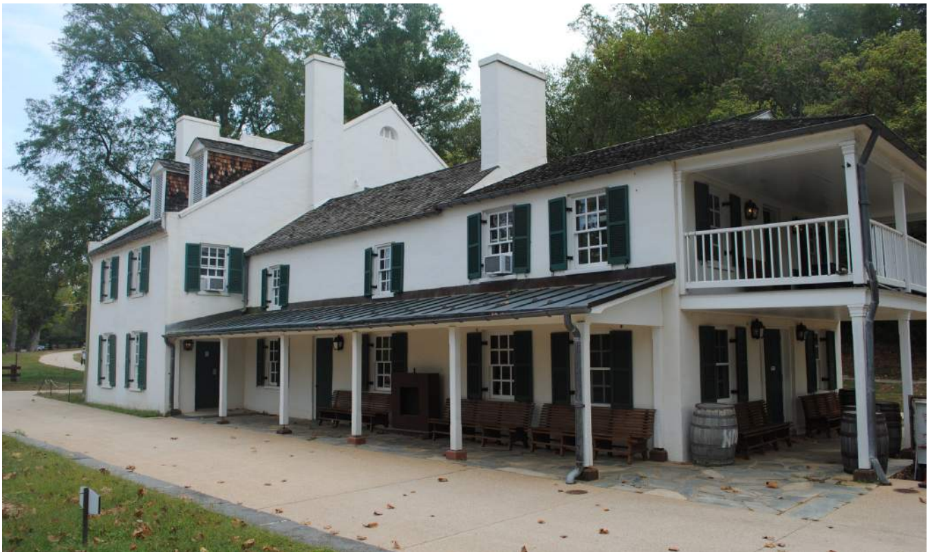
Figure 119: West Elevation Looking Northeast (BBB 2019)
