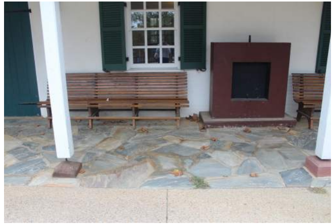
Figure 166: Flagstone Paving and Slab on Grade in West Porch (Silman 2019)
