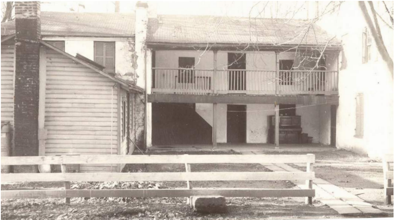
Figure 39: East Elevation with Frame Kitchen Addition, 1939. (CHOH NHP)
