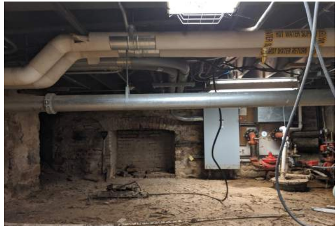
Figure 125: South Wing Cellar Looking Southeast (BBB 2019)
