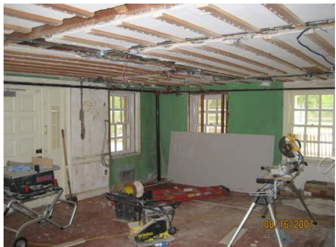
Figure 104: Interior of South Wing First Floor During Renovation, August 16, 2007. (NPS)
