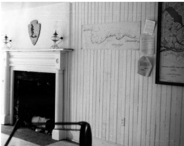
Figure 88: South Wing, Second Floor After Renovation, North Wall Looking Northwest, ca. 1970s. (CHOH NHP)
