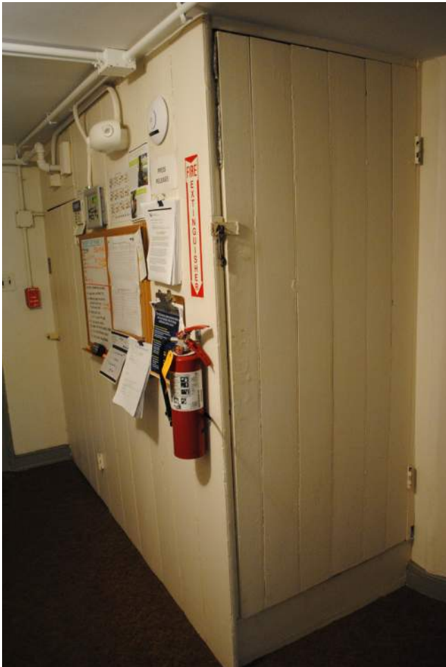
Figure 146: North Wing, Second Floor Hall Looking Southwest to Attic Stairs (BBB 2019)
