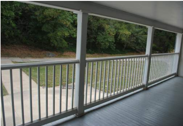
Figure 117: East Elevation, Second Story Porch Looking Southeast (BBB 2019)
