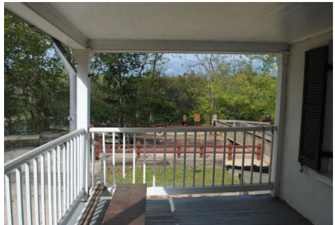
Figure 120: South Porch, Second Story Looking West (BBB 2019)
