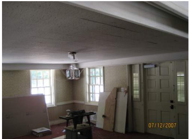
Figure 103: Interior of South Wing First Floor Before Renovation, July 12, 2007. (NPS)
