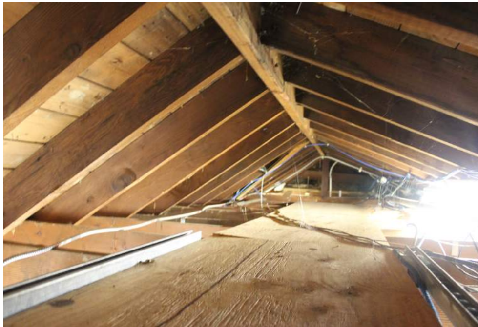
Figure 173: Center Section Roof Framing Looking Above Collar Joists (Silman 2019)
