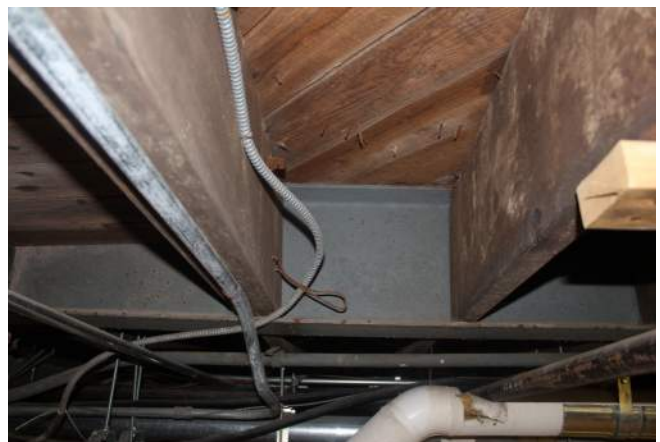
Figure 168: Joist Bearing on Steel Beam in South Wing (Silman 2019)
