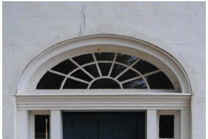
Figure 186: Historic Fanlight Above Main Entrance, North Elevation (BBB 2019)
