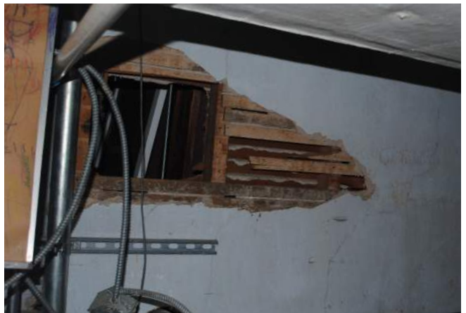
Figure 188: Historic Wood Lath and Plaster in Third Floor (BBB 2019)
