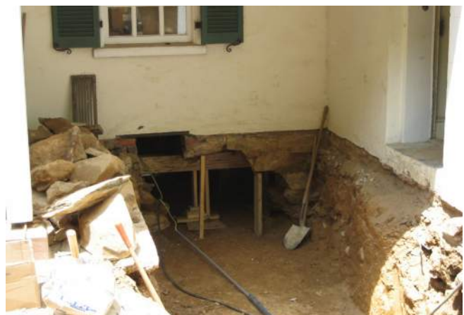
Figure 93: Excavation and Shoring Cellar Beneath Center Section, East Elevation, June 12, 2007. (NPS)
