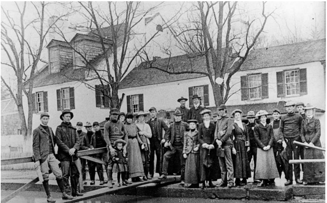
Figure 26: Group at Lock 20 in Front of West Elevation, ca. 1900. (Canal Trust)
