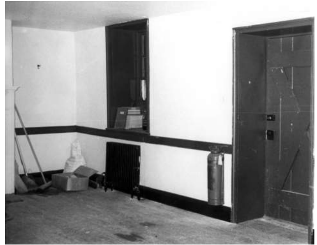
Figure 65: Center Section, First Floor During Renovation, Northeast Corner Looking Northeast, ca. 1950s. (CHOH NHP)
