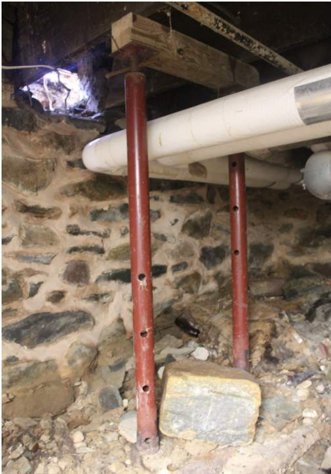
Figure 170: Cellar Shoring Posts (Silman 2019)
