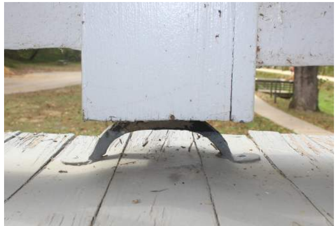
Figure 163: South Porch Post Base at Second Floor (Silman 2019)
