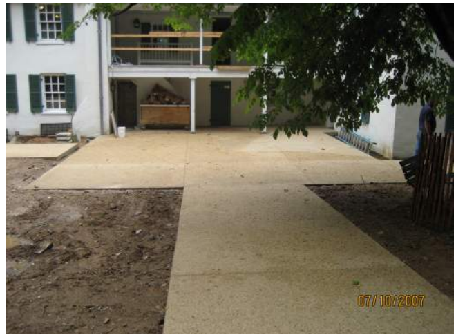
Figure 97: New Concrete Walkways at East Elevation, July 10, 2007. (NPS)
