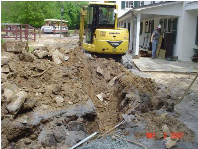
Figure 96: Demolition Work West of Tavern, May 3, 2007. (NPS)
