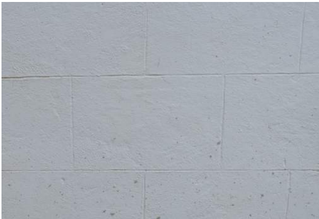
Figure 185: Scored Stucco on North Wing (BBB 2019)
