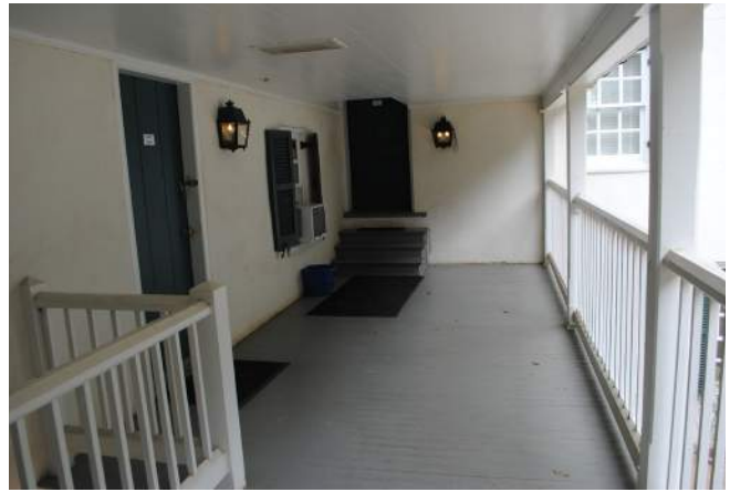
Figure 116: East Elevation, Second Story Porch Looking North (BBB 2019)
