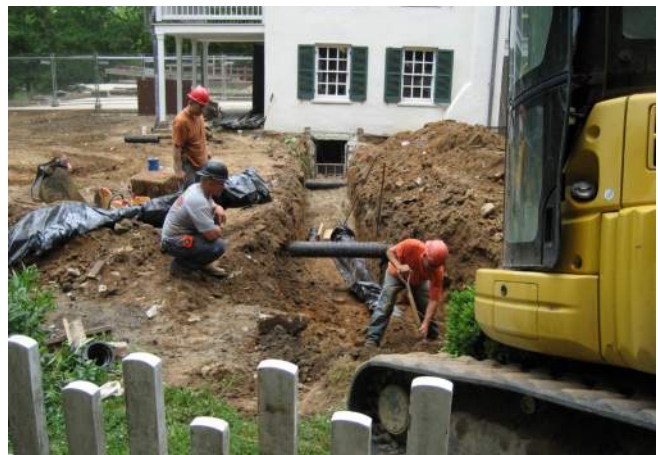
Figure 92: Installing Utility Trench at East Elevation, June 5, 2007 (NPS)
