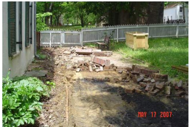
Figure 91: Removing Brick Walkways at East Elevation, May 17, 2007. (NPS)
