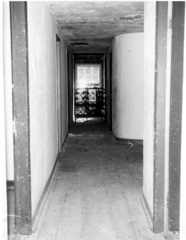
Figure 57: North Wing, Second Floor Before Renovation, Main Hallway Looking East, ca. 1950s. (CHOH NHP)
