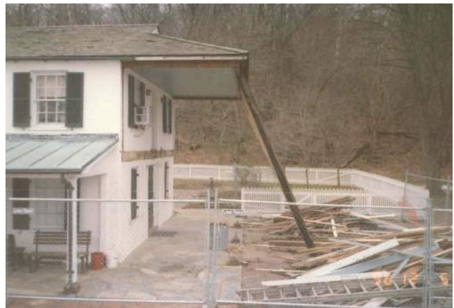
Figure 90: South Porch Structure Removed, December 12, 1996. (NPS)
