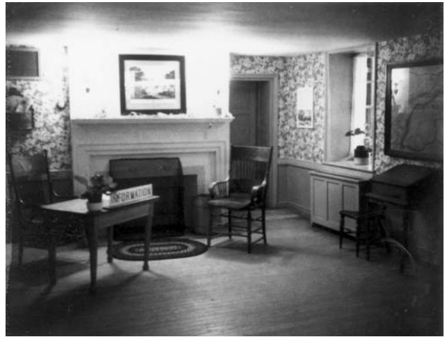
Figure 79: North Wing, First Floor After Renovation, Southwest Corner Southwest, ca. 1970s. (CHOH NHP)
