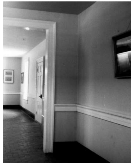
Figure 55: North Wing, First Floor, Looking Southeast to Opening Perpendicular to South Wall, ca. 1951. (CHOH NHP)
