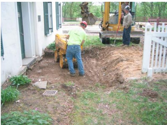
Figure 98: Regrading Front Walkway, May 3, 2007. (NPS)
