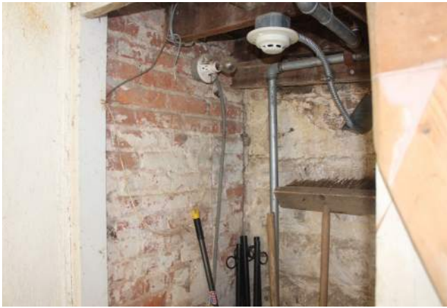
Figure 161: Brick and Stone visible from Closet Below East Porch (Silman 2019)
