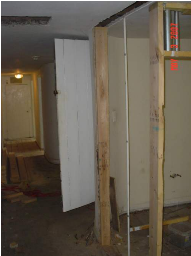
Figure 105: Constructing Bathroom at North Wing Second Floor, Looking Southeast, May 3, 2007. (NPS)
