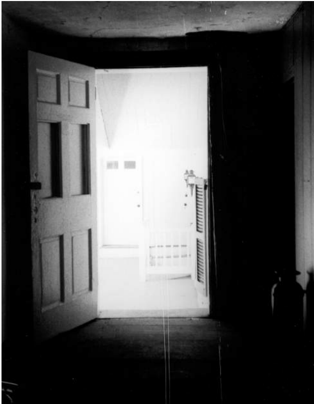
Figure 56: North Wing, Second Floor Before Renovation, Door in South Wall Looking South, ca. 1950s. (CHOH NHP)
