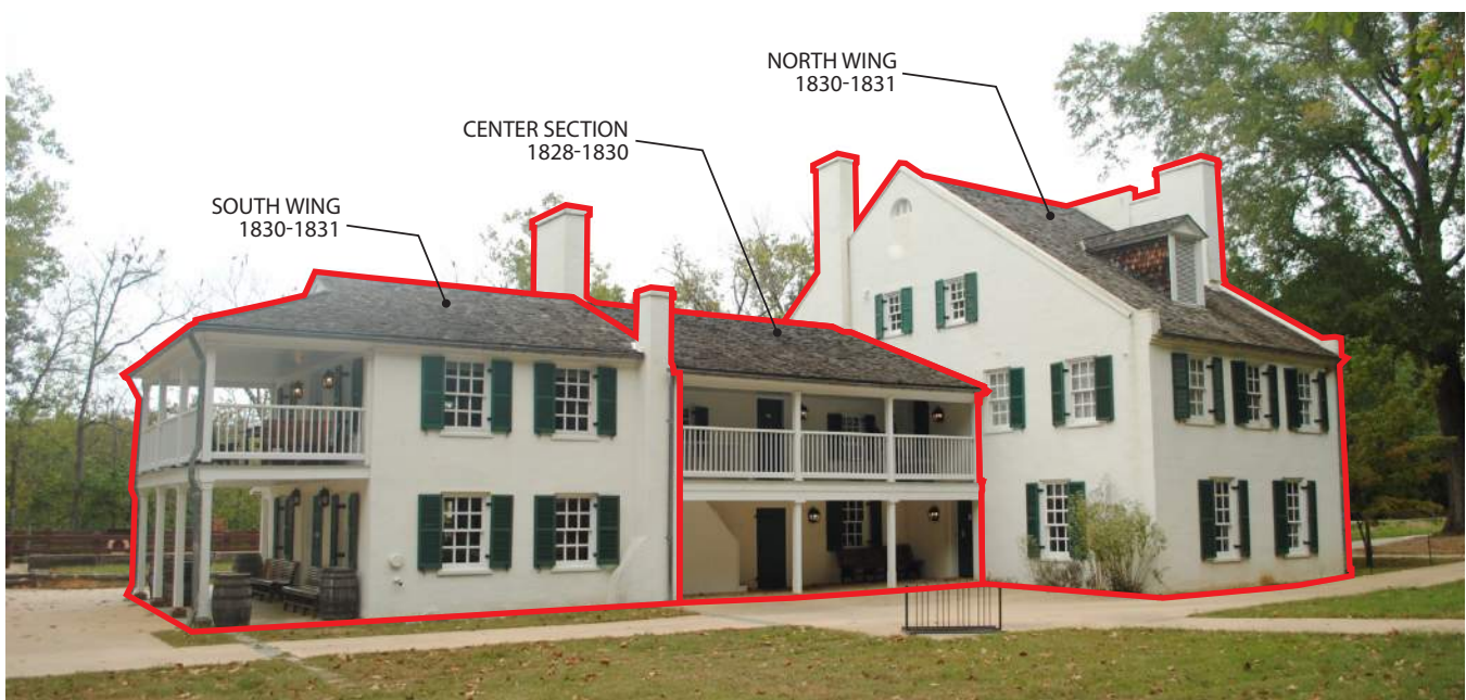
Figure 108: Building Key; East Elevation Showing South Wing (Left), Center Section (Middle), and North Wing (Right) (BBB 2019)
