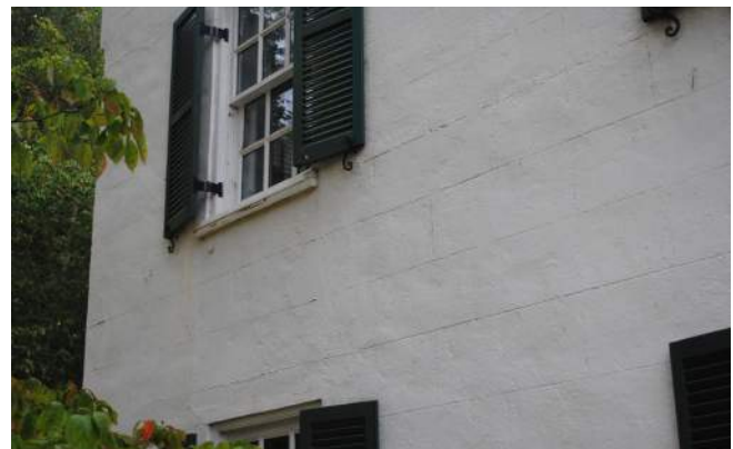
Figure 110: Detail of North Elevation Showing Scored Stucco (BBB 2019)
