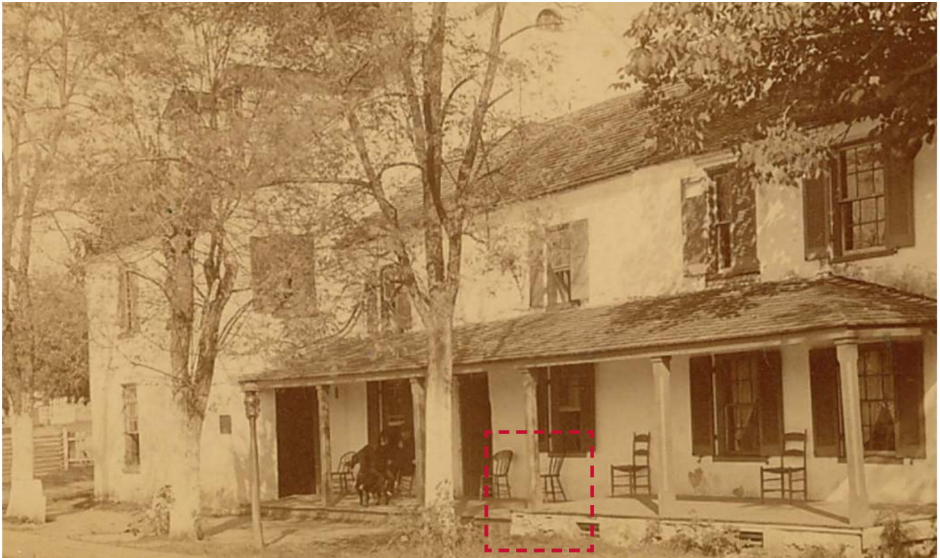
Figure 21: West Elevation with West Porch, 1889. Note change in floor level of porch identified in red. (Montgomery County Historical Society [MCHS])
