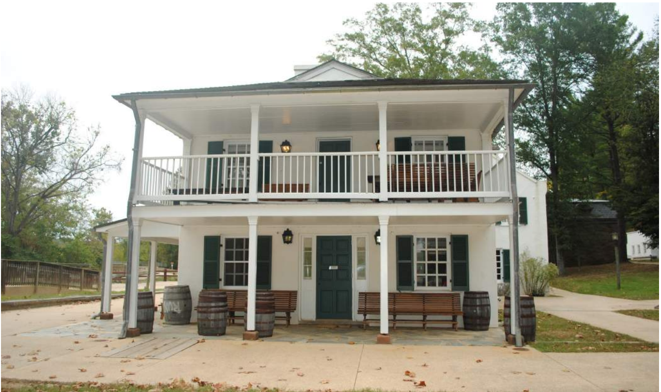
Figure 121: South Elevation Looking North (BBB 2019)
