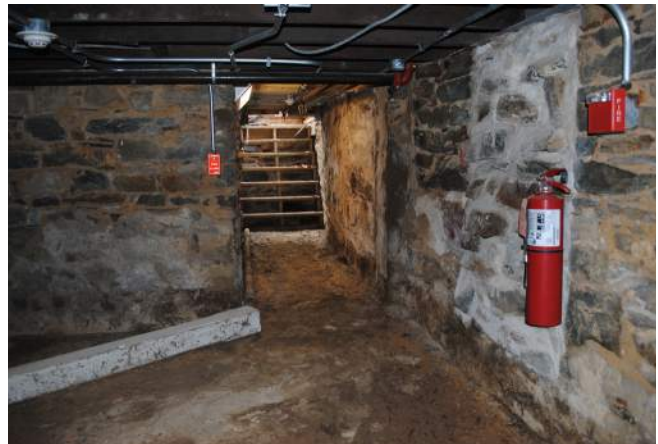
Figure 126: South Wing Cellar Looking Southwest to Entrance Stairs. (BBB 2019)
