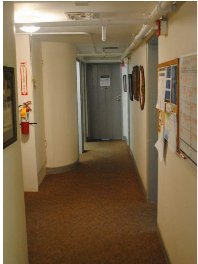
Figure 141: North Wing, Second Floor Hallway (Rm 201) Looking West (BBB 2019)
