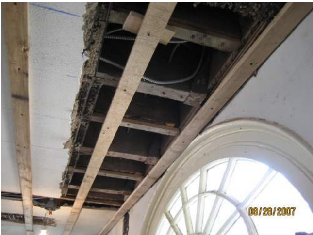
Figure 100: Interior of North Wing First Floor During Renovation, August 28, 2007. (NPS)
