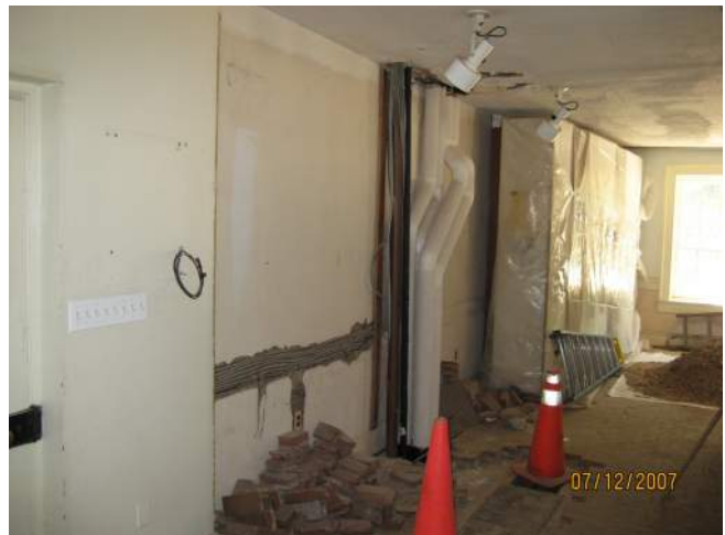
Figure 101: Interior of North Wing First Floor During Renovation, July 12, 2007. (NPS)
