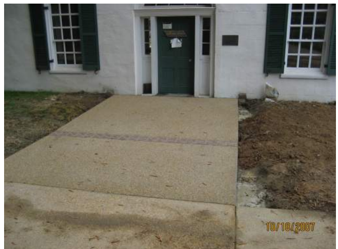
Figure 99: After Front Walkway Regraded, October 18, 2007. (NPS)
