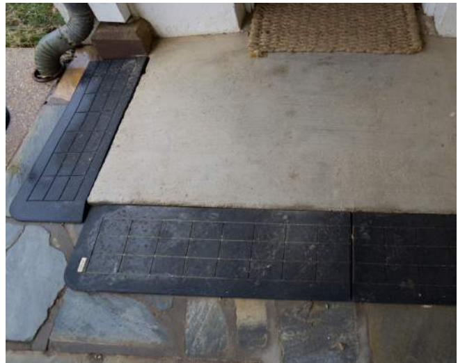
Figure 176: Temporary ramp at exterior concrete pad at Door 101A (BBB 2019)
