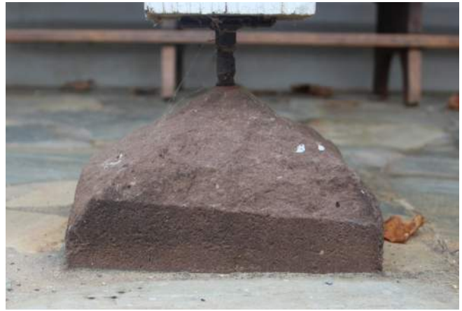
Figure 162: West Porch Post Base at Grade (Silman 2019)
