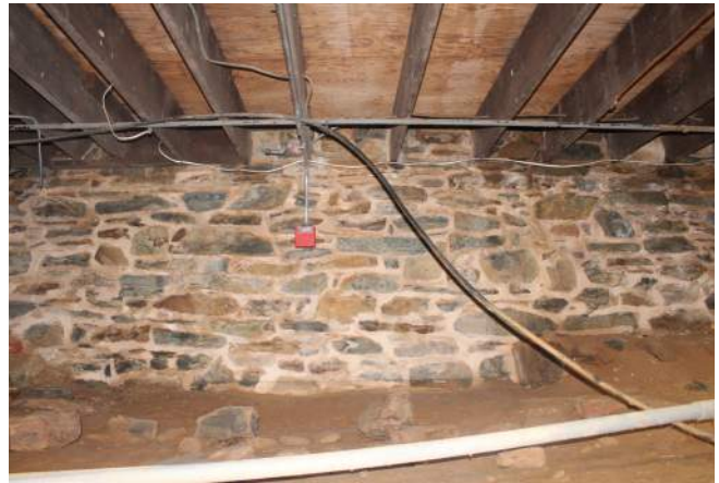
Figure 167: Center Section Joist Framing; Likely 1949 Restoration (Silman 2019)
