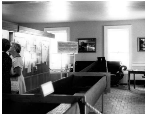
Figure 53: North Wing, First Floor After Renovation, West Wall Looking Southwest, ca. 1951. (CHOH NHP)
