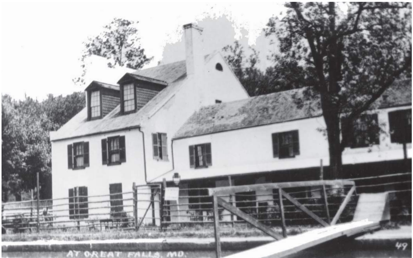
Figure 36: West Elevation, Looking Northeast from Lock 20, ca. 1913. (CHOH NHP)
