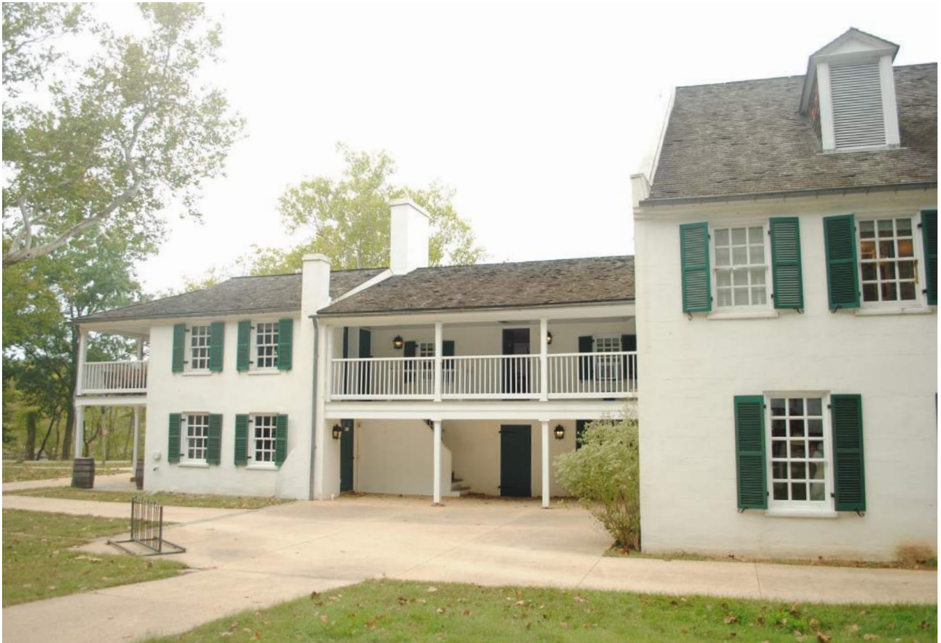
Figure 113: East Elevation Looking Southwest (BBB 2019)
