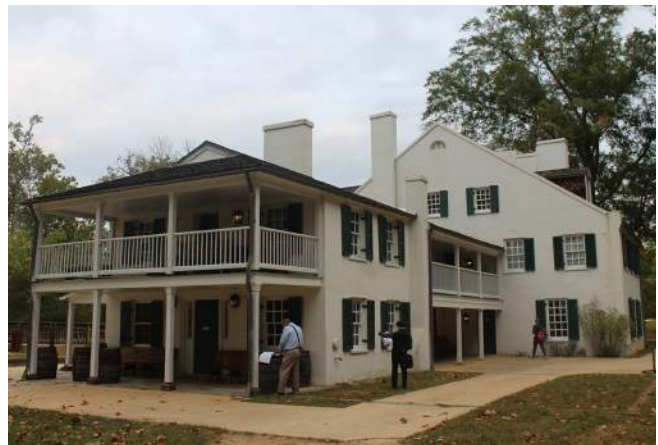
Figure 158: Great Falls Tavern Viewed from the Southeast (Silman 2019)
