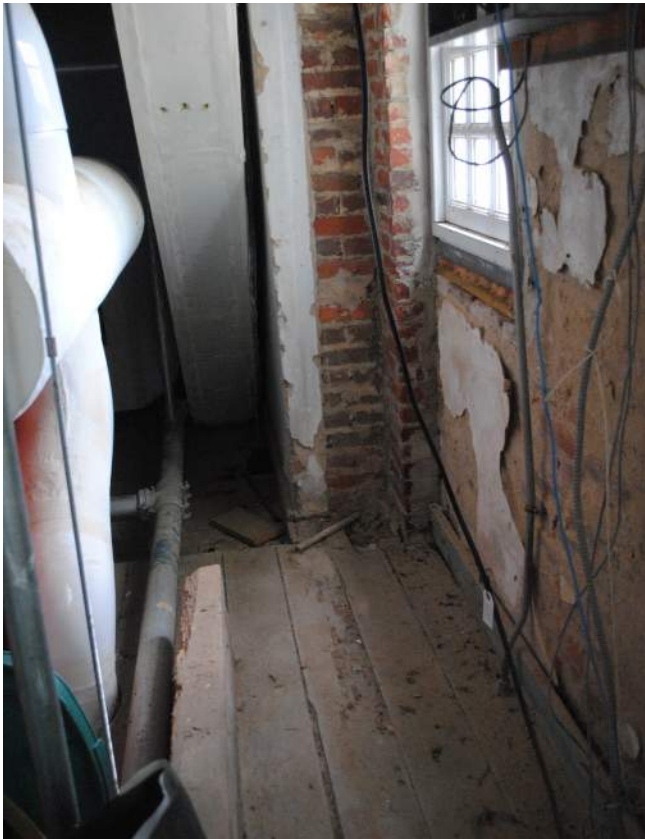
Figure 155: North Wing Attic Exterior Wall and Floor, (BBB 2019)
