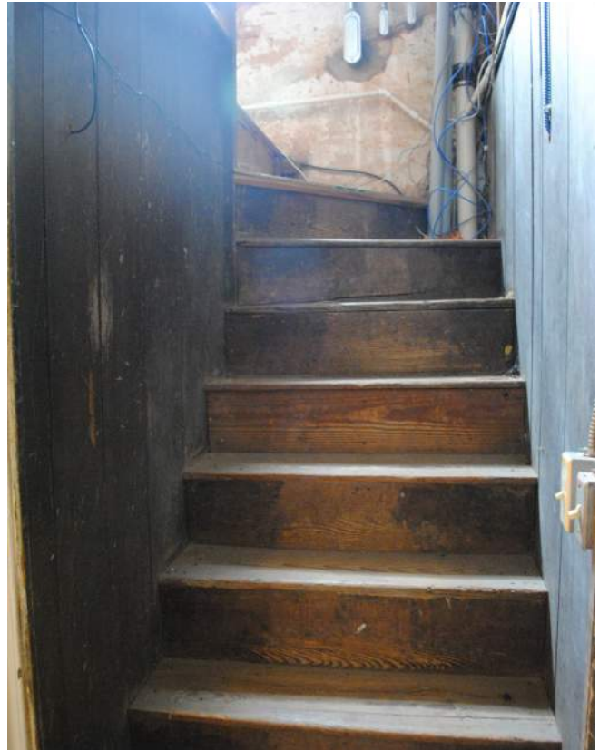
Figure 156: North Wing Attic Stairs Looking South from Second Floor Hallway (BBB 2019)
