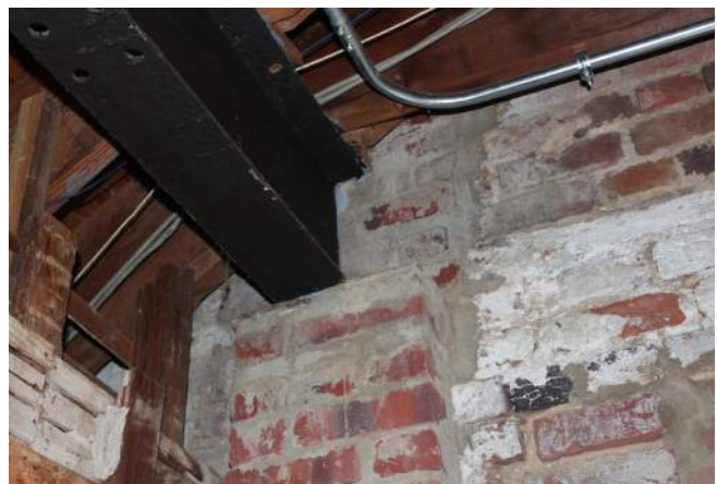
Figure 171: Steel Beam Supporting North Wing Attic (Silman 2019)
