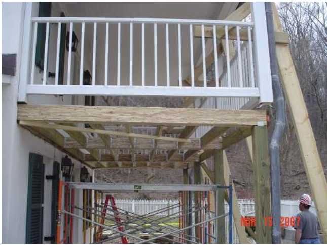
Figure 94: Reconstructing South Porch, March 15, 2007. (NPS)
