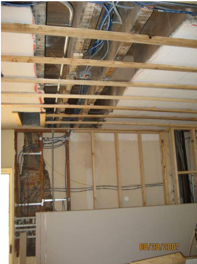
Figure 102: Interior of North Wing First Floor During Renovation, August 28, 2007. (NPS)
