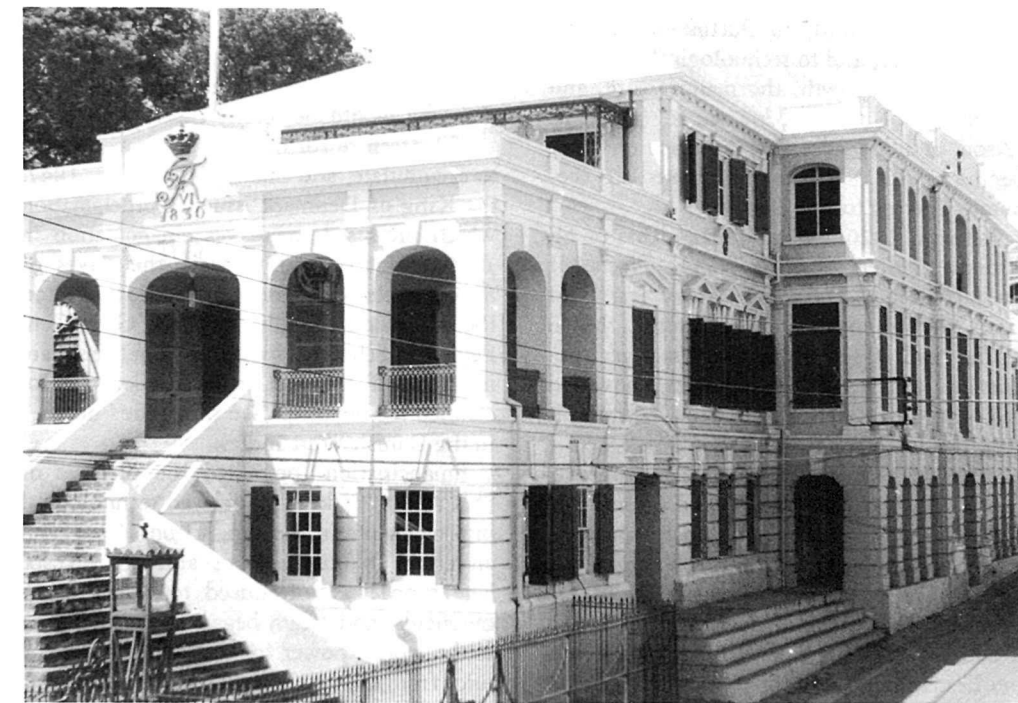
Government House, an 18th-century structure with 19th-century additions.
