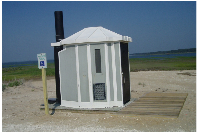
Top: Climate change scenario planning workshop in the NPS Alaska Regional office. Bottom: Sustainable park infrastructure at Assateague Island National Seashore is designed for a barrier island where sea level rise and increase storm frequency are projected. Vault toilet mounted on a wooden deck to allow easy relocation during storm events.
