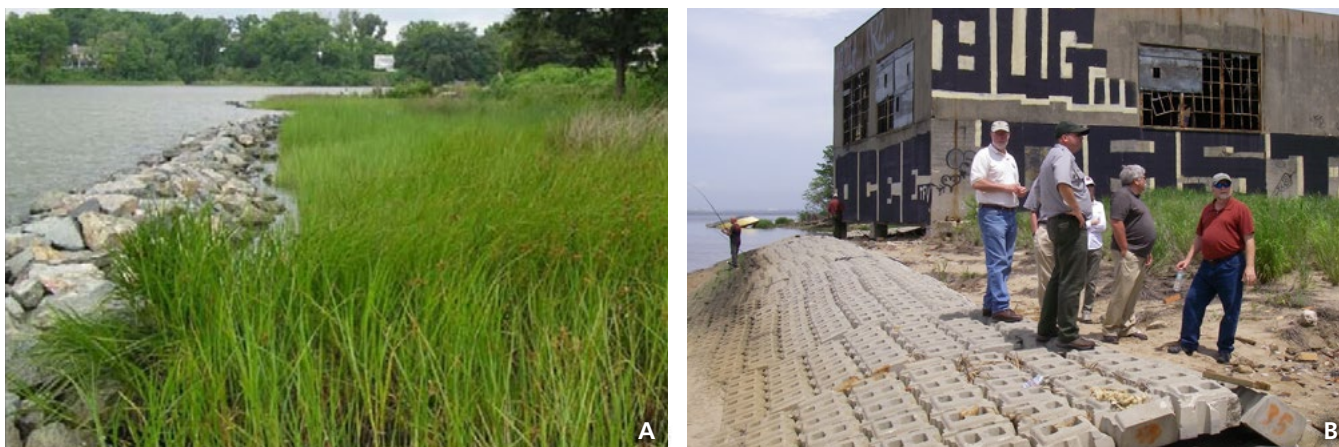
Figure 8.7. Examples of hybrid approaches to living shorelines. Notes: (a) This hybrid approach to a living shoreline uses natural and nature-based features by combining a planted marsh with a rock sill. Photograph from Bilcovic and Mitchell (2011). (b) The vegetation component of this hybrid approach at GATE was unsuccessful, leaving only shoreline armoring. Photograph by NPS.
