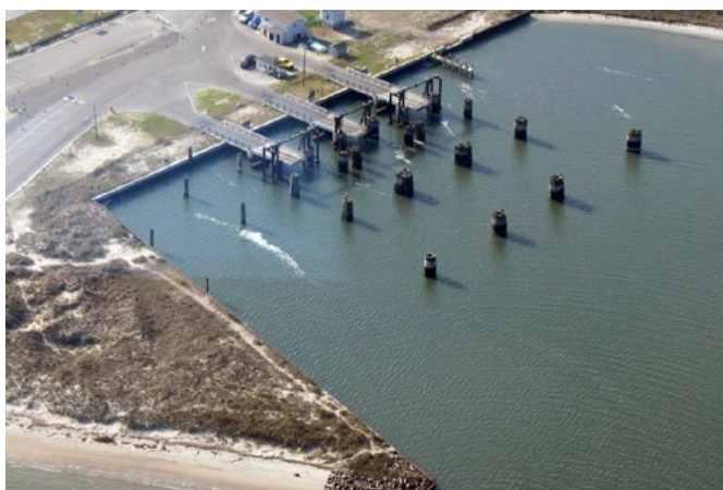
Figure 8.3A. Bulkheads at the Hatteras Island ferry landing on Ocracoke Island, NC. Photograph by NPS.
