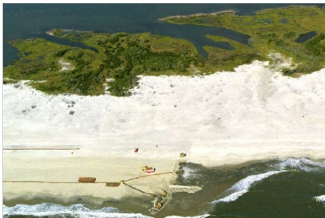
Figure 8.6. Beach nourishment at Assateague Island National Seashore in 2002 added sediment and widened the beach. Photograph by NPS.
