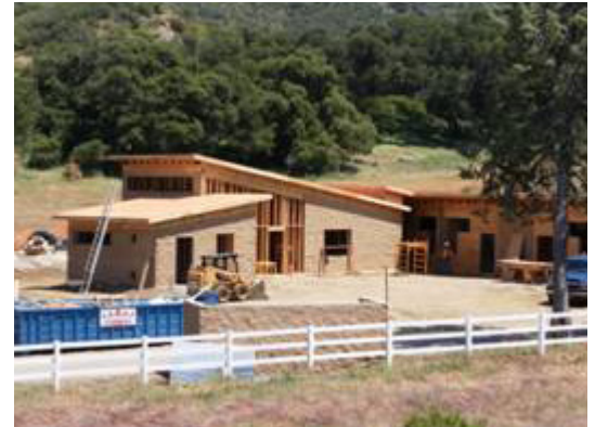
Intern Center under construction - April 2010. Photo courtesy of Kim Park.
