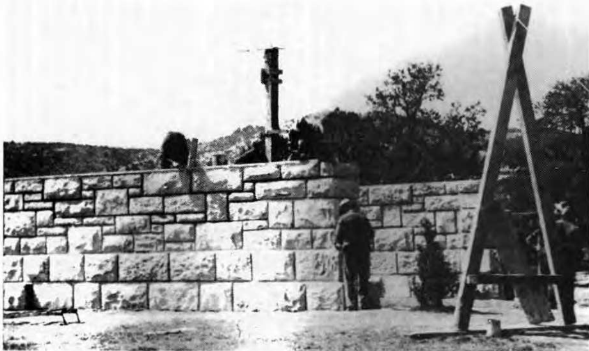
Constructing stone walls on the Colorado National Monument.
