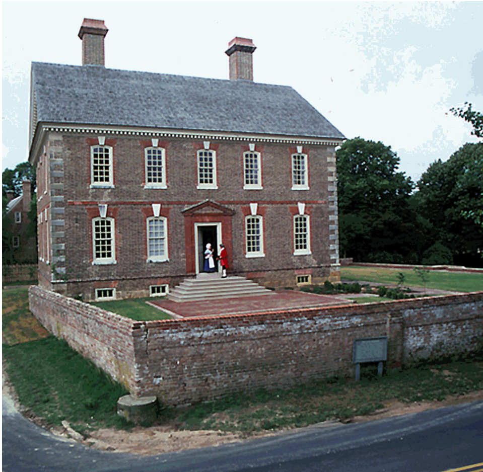
Figure 12. The recently restored Nelson House with its front court showing the new steps, walks, and boxwood hedge, ca. 1976. The perimeter brick wall had not yet been lowered (Richard Freer, National Park Service, Harpers Ferry Center).
