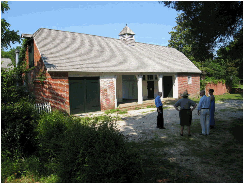
Figure 14. The service drive and stable looking west, June 2007 (SUNY ESF).
