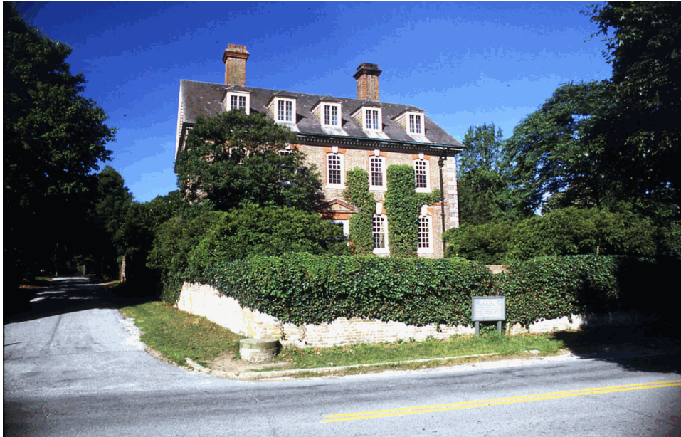
Figure 11. The Nelson House and lowered boxwood hedge, looking south across Main Street, June 1972 (Richard Freer, National Park Service, Harpers Ferry Center).
