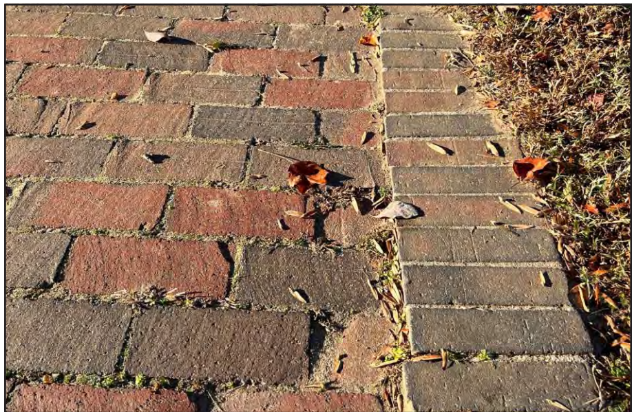
Figure 4.15 Existing brick walks at the terrace are from the NPS management era. The soldier course edging could be a tripping hazard.
