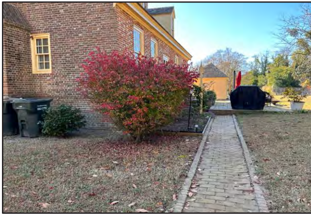
Figure 2.11 (top). The Smith House looking northwest from Nelson Street, 2023.
