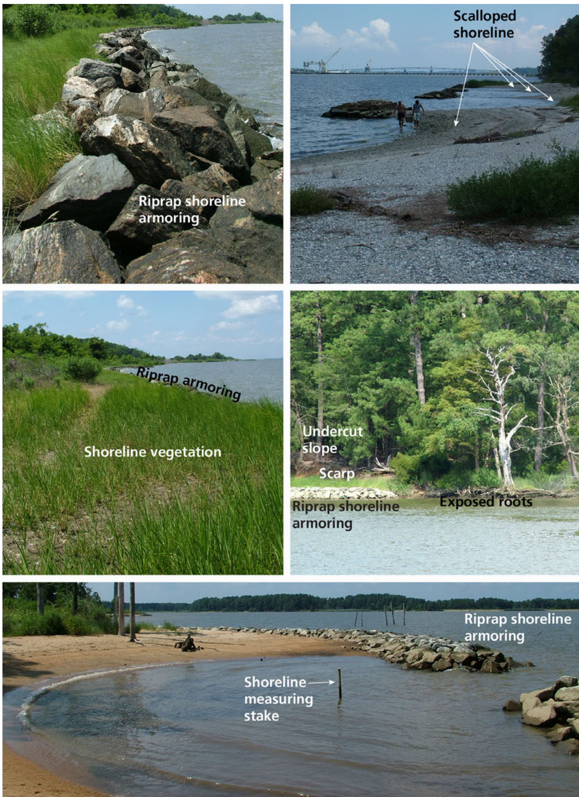
Figure 22. Photographs of shoreline stabilization structures. Riprap and artificial fill (geologic map unit Qf) were installed on many shorelines within the park. In some places, vegetation is able to grow behind the riprap, in others, refracted waves cause erosion behind the structure. National Park Service photographs taken by Melanie Peters (NPS Geologic Resources Division) in August 2005.
