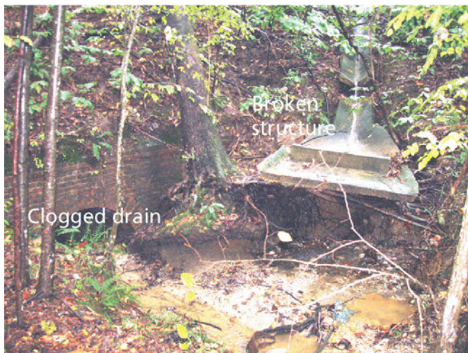
Figure 27. Photographs of stormwater management structures along the Colonial Parkway. Many of the culverts and drains within the park are inadequate to handle the flow following common heavy precipitation. Structures are many decades old, cracked, and/or clogged. As impervious surfaces increase with urban development, more runoff is anticipated in the future. National Park Service photographs taken by Harold Pranger (NPS Geologic Resources Division) 28 September 2004.
