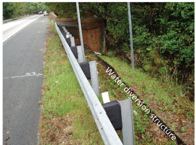
Figure 27. Photographs of stormwater management structures along the Colonial Parkway. Many of the culverts and drains within the park are inadequate to handle the flow following common heavy precipitation. Structures are many decades old, cracked, and/or clogged. As impervious surfaces increase with urban development, more runoff is anticipated in the future. National Park Service photographs taken by Harold Pranger (NPS Geologic Resources Division) 28 September 2004.
