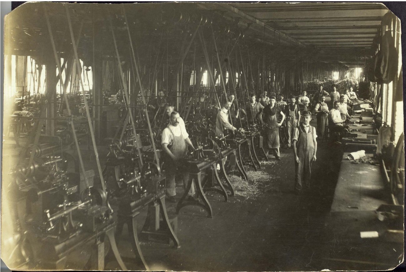
Colt employees on the shop floor, circa 1900, courtesy of the Connecticut State Library
