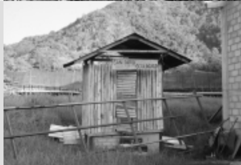
Composting latrine built from indigenous materials
