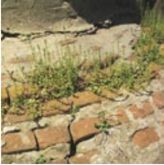
Top: A foaming test treatment is applied to vegetation growing at Castillo de San Marcos National Monument, the oldest masonry fort in the continental United States.
