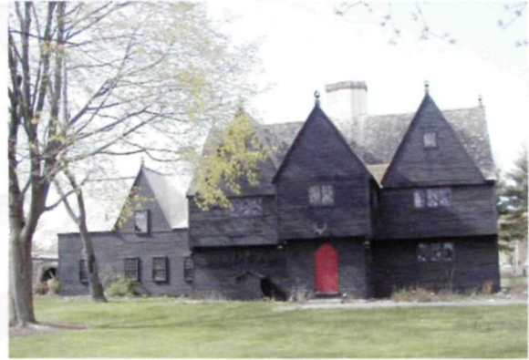
Ironworks House (17th Century), Saugus Ironworks National Historic Site.
