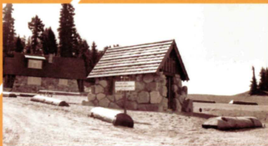
Entrance station at the North Junction, with a ranger residence in the background, 1936. Buried logs were intended for traffic control.
