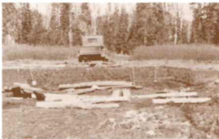
Crews dug peat from bogs near Park Headquarters as soil amendment for planting along the Rim Drive, 1934.
