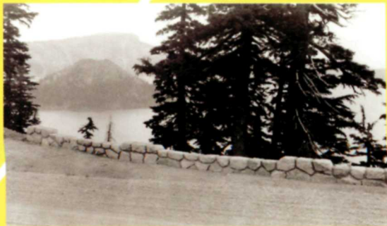
The masonry guardrail built along Rim Drive was very carefully planned to enhance the view.
