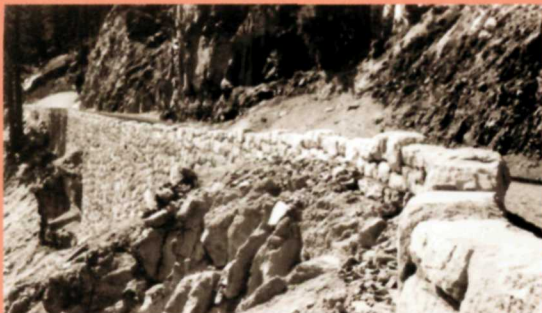
A retaining wall at the base of Dutton Cliff measuring more than fifty feet high, 1939.
