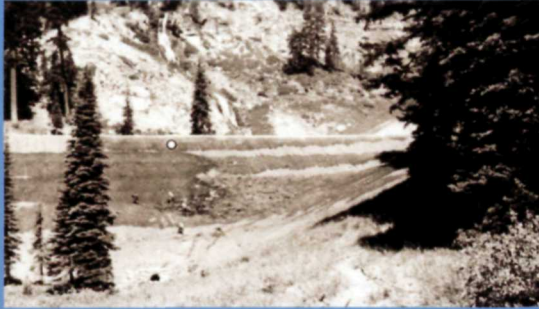
In 1939 workers planted a massive fill that served to bridge the creek below Vidae Falls.
