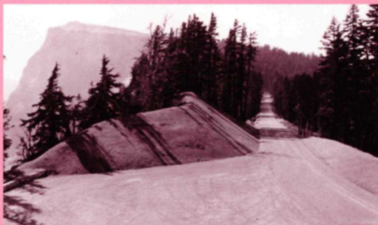
Newly completed bank slope built at a point overlooking Steel Bay, 1936.
