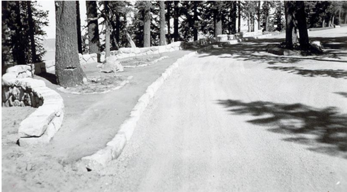
History #6: Parking area associated with the Kerr Notch observation station. Note curbing, guard walls and planting beds visible in photo, 1938 (Lange, CLNPMAC).
