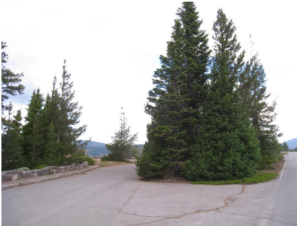
Circulation #10: View of Grotto Cove substation (Germano, PWR, 2010).
