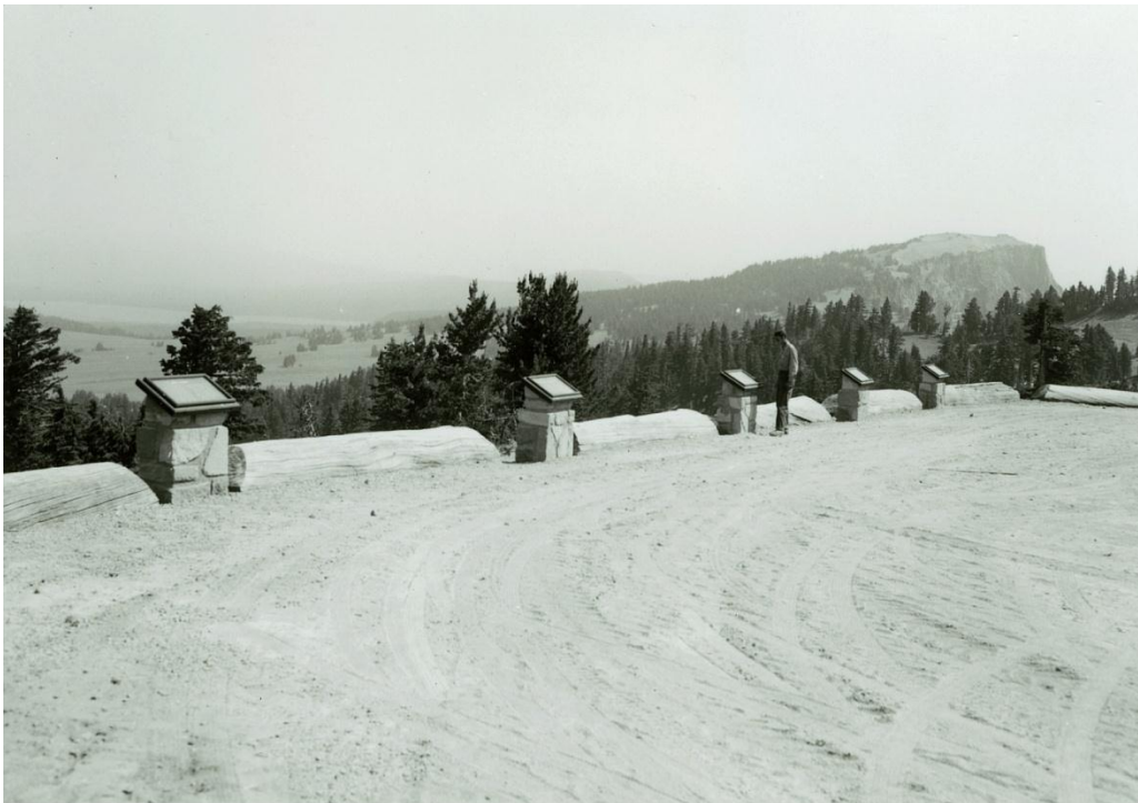
History # 10: The Diamond Lake substation with wayside exhibits located between log guardrails, 1959 (CLNPMAC).
