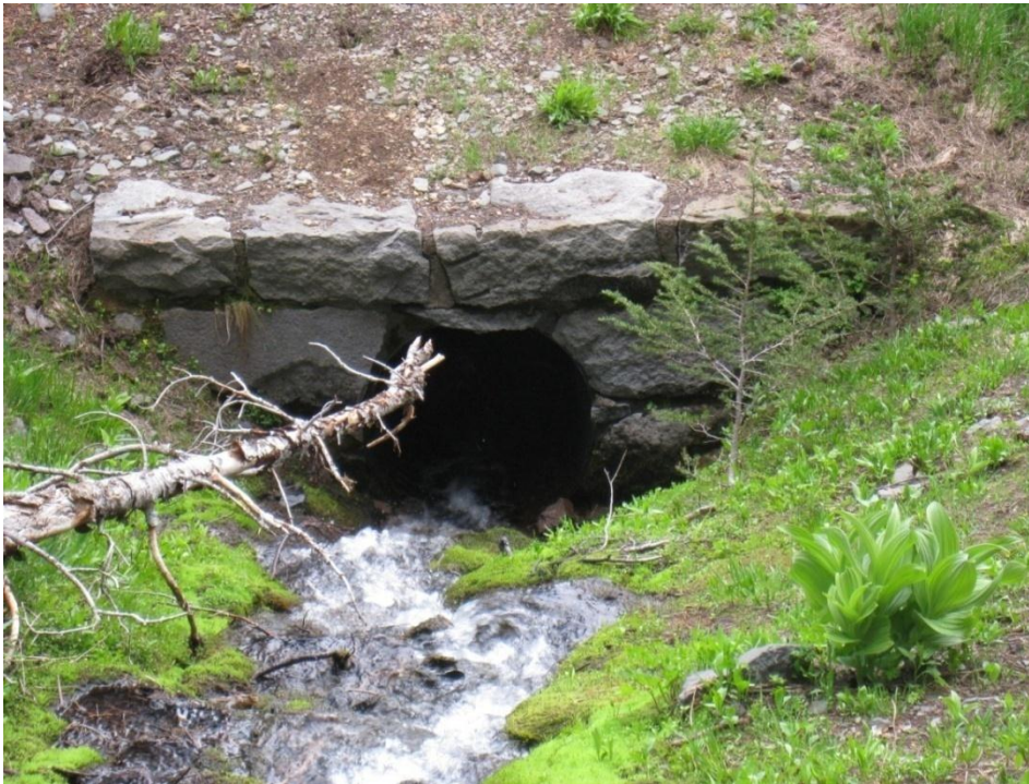
Buildings and Structures #6: Culvert with stone masonry headwall near Sun Creek Valley Vista (Gjesfjeld, PWR, 2010).
