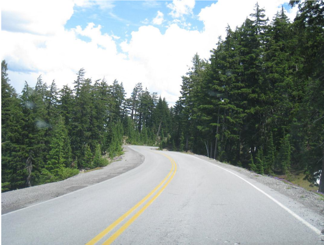
Circulation #3: View of Segment 7-B of Rim Drive at approximately mile 7.4 (Germano, PWR, 2010).
