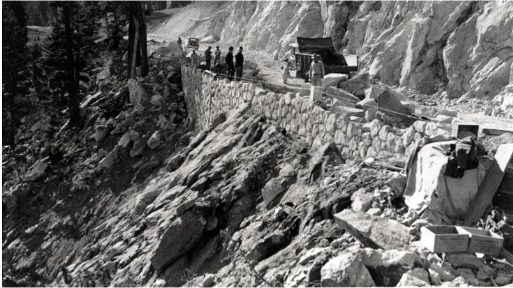
History #3: Construction of a stone masonry retaining wall at Scott Bluffs, 1934 (Doerner, NARA, RG 79, SB).
