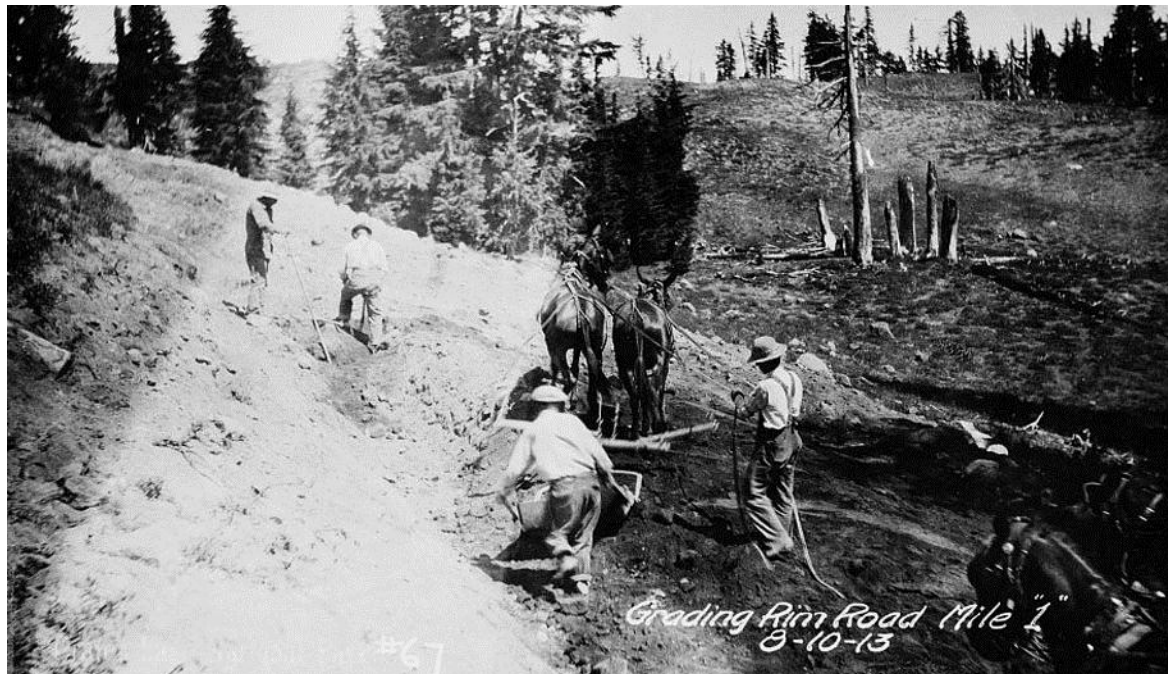
History #1: Grading the old Rim Road, 1913 (NARA, RG 77, DC).
