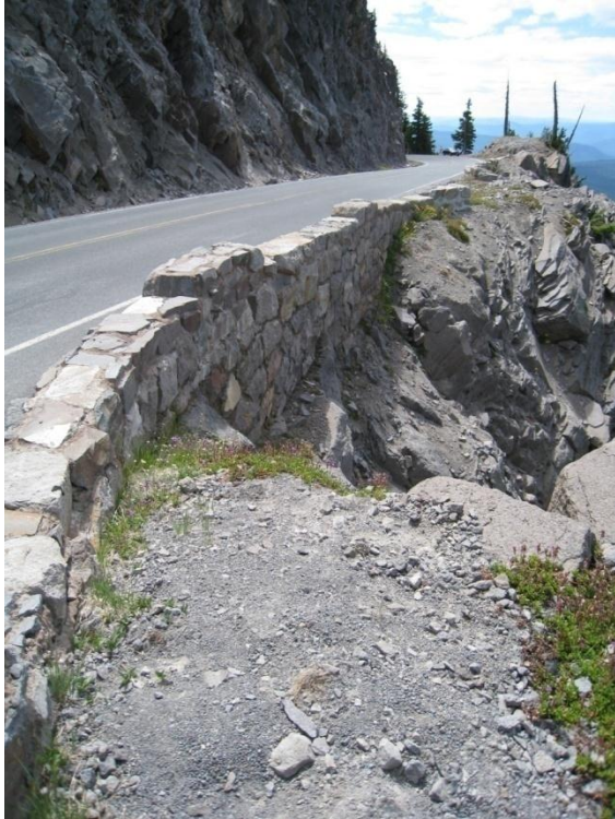
Buildings and Structures #3: Stone masonry retaining wall and guardrail along Rim Drive (Hartzler, PWR, 2008).
