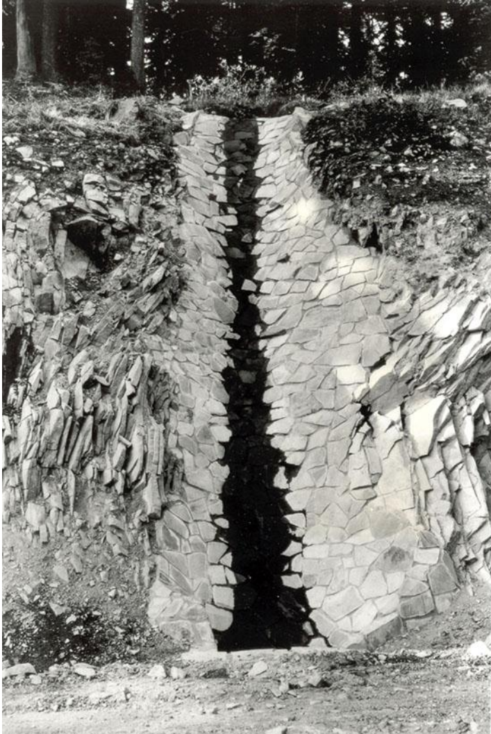
History #8: Stone masonry spillway located along segment 7-D2 (Lange, NARA, RG 79, SB).
