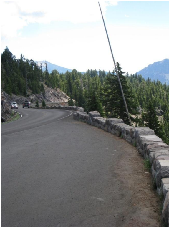
Buildings and Structures #2: Curvilinear stone masonry guard wall at Union Peak substation (Gjesfjeld, PWR, 2010).
