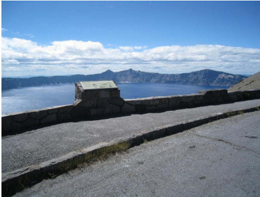
Buildings and Structures #1: View of Crater Lake from Cloudcap observation station. Note the interpretive sign, stone masonry wall and curbing in the foreground (Hartzler, PWR, 2008).
