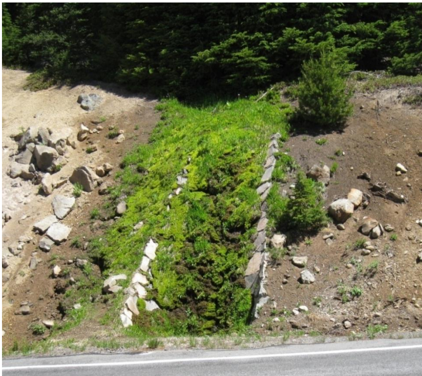
Buildings and Structures #4: Stone masonry spillway overgrown with moss and grass along Rim Drive segment 7-D (Gjesfjeld, PWR, 2010).
