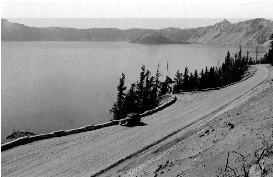
History #4: Parking area and associated guard wall near Cleetwood Cove in segment 7-B, 1936. Note the merlons and curvilinear form of the guard wall (Lange, NARA, RG 79, SB).
