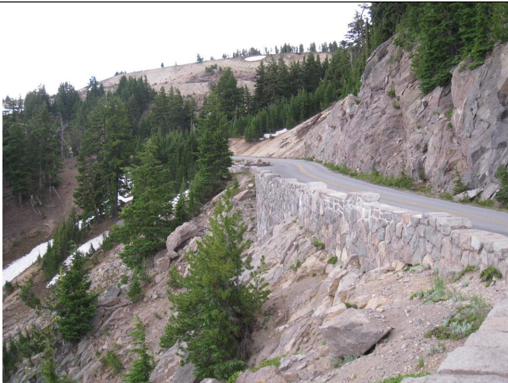
Circulation #5: View of Segment 7-C of Rim Drive at approximately mile 15.1 (Germano, PWR, 2010).
