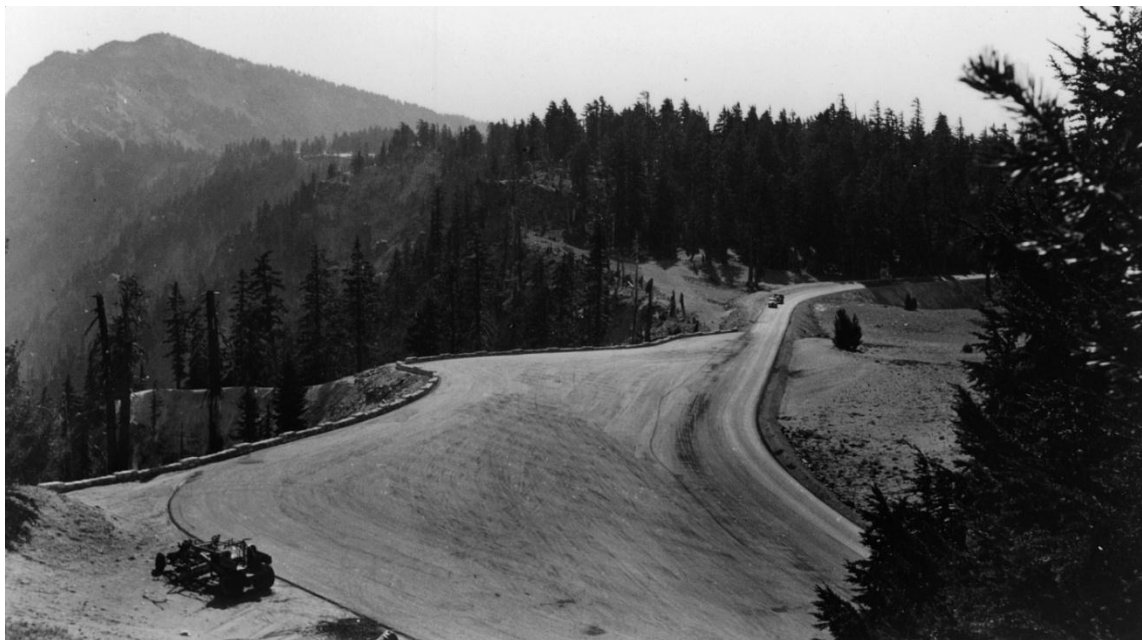
History #5: Parking area near Discovery Point. Note masonry guard wall with merlons, 1935 (Lange, NARA, RG 79, SB).
