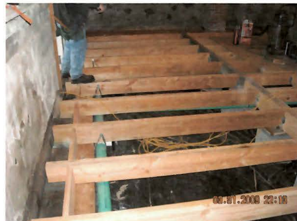
New floor joists to replace rotten flooring system
