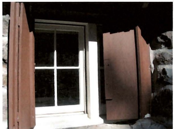
Bi-fold plywood permanent shutters
