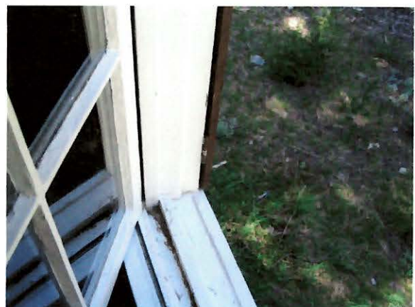
Window frame detail
