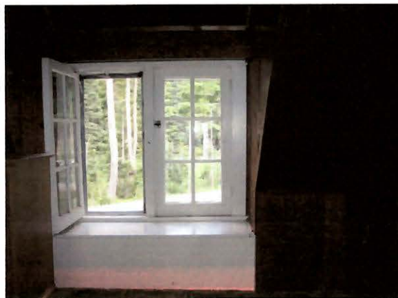
Dormer facing East
