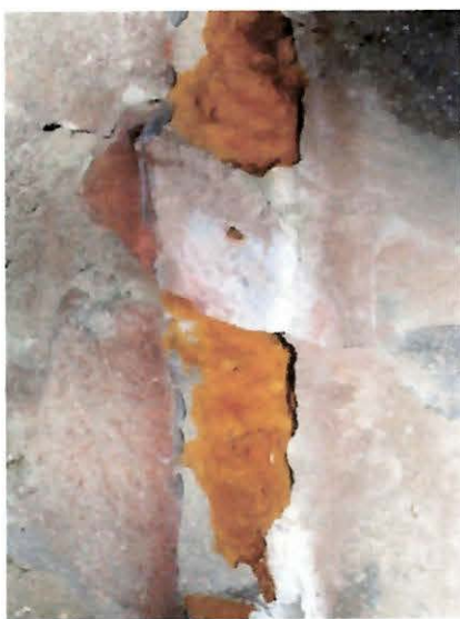
Spray foam in masonry joint
