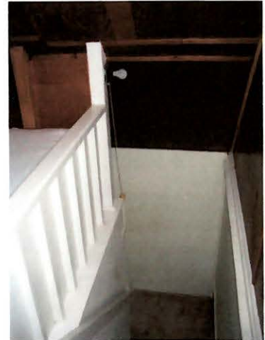
Stairway detail facing West
