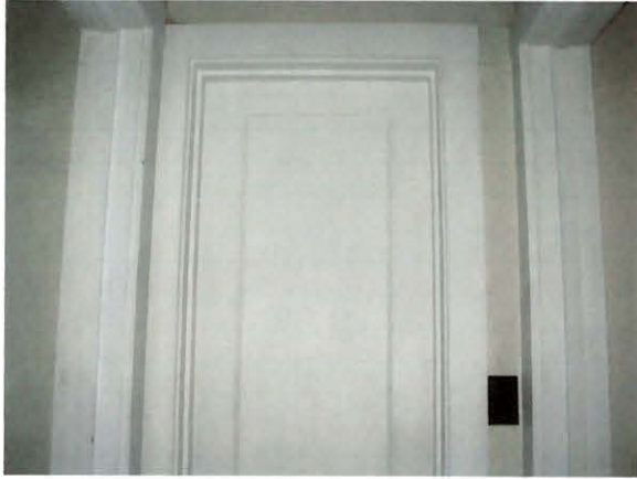
Bathroom door and bedroom door frames
