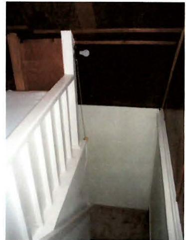
Stairway detail facing West
