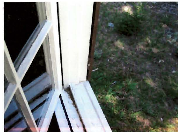
Window frame detail
