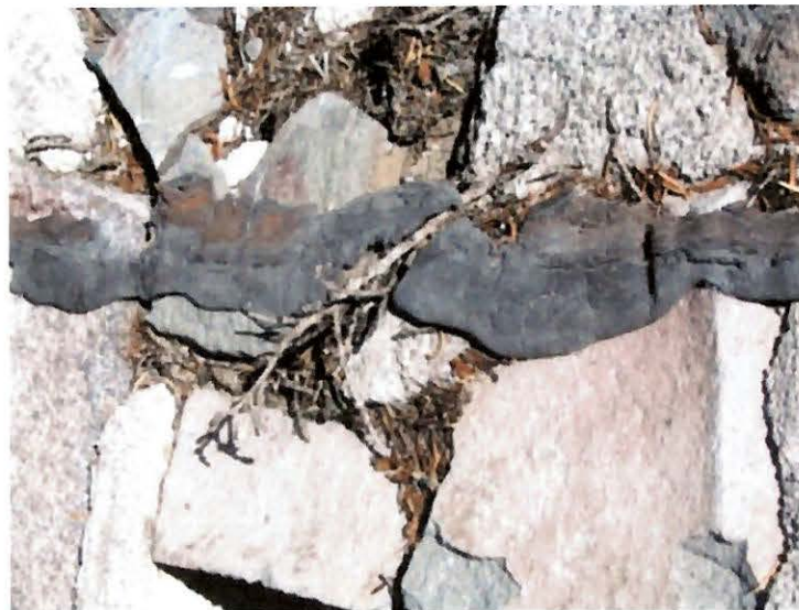
Black silicone used for attaching snow tunnels on patio wall
