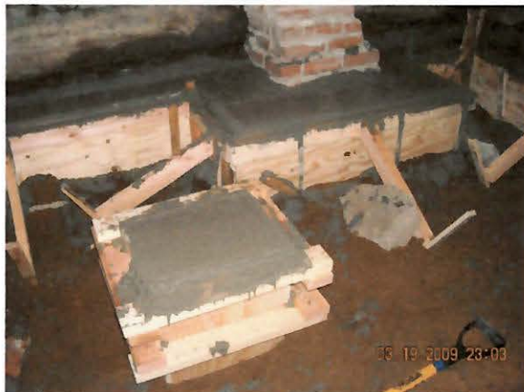
New concrete pier and stem-wall foundation
