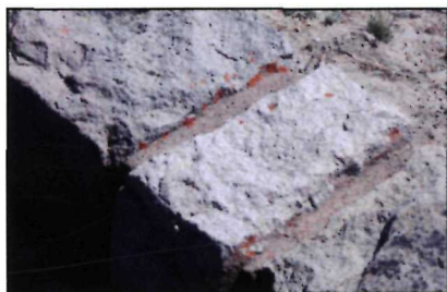
The guard wall at the turnout at mile 10.5 shows the red tint found in historic mortar.
