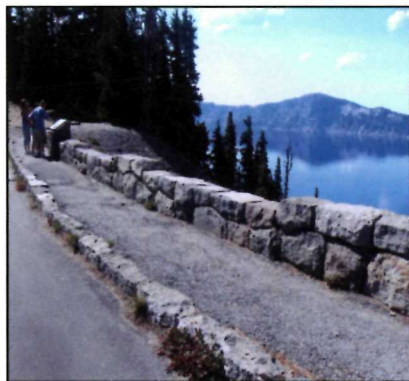
Guard wall at Pumice Castle Overlook at mile 11.0 showing proper variation in stone size, shape, and color.
