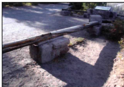
Stone masonry pier and log guard rail at the Pinnacles Overlook.
