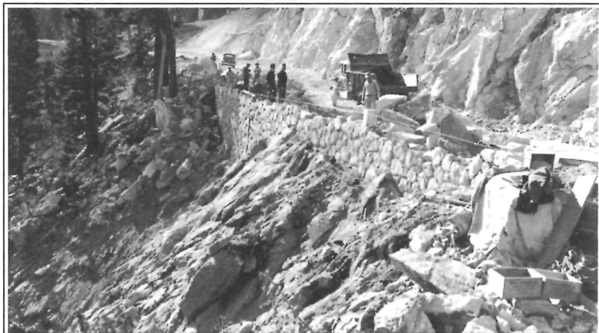
Historic photograph of stonemasons building a retaining wall at Scott Bluffs, 1934 (Photo: National Park Service)
