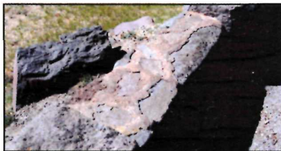
Guard wall at Sentinel Point (mile 10.7), showing incompatible repair.
