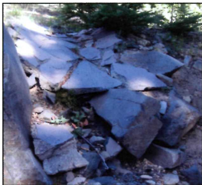
Deterioration of a tiled masonry drain across from the Sun Notch parking lot at mile 4.4
