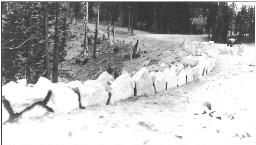
Historic photograph of the construction of a stone masonry guard wall near Pumice Point, 1934 (Photo: National Park Service)
