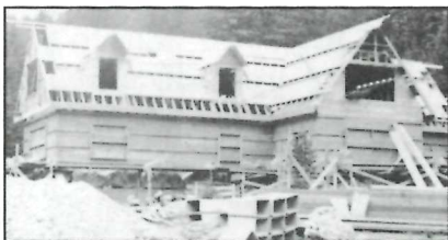
Construction of the Superintendent's Residence showing application of the exterior layer of masonry (Photo: National Park Service).
