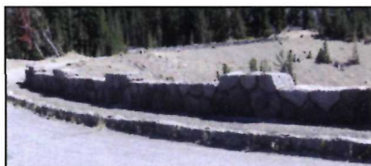
Guard wall at mile 15.8 showing merlons and curvilinear form.
