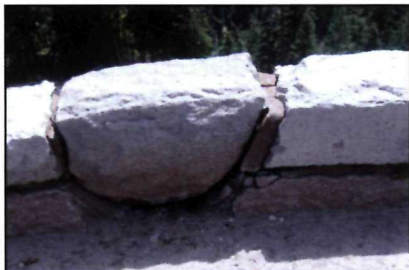
Guard wall at mile 4.5-5.0 on Sun Grade showing a loose stone caused by mortar deterioration.
