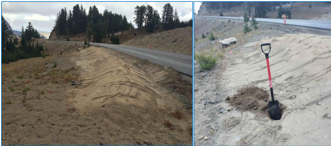
Figure 18. An obliterated pullout with insufficient site preparation, as the restored area looks more like a “worm” of placed topsoil rather than a natural landscape feature (left). Checking for soil compaction in a recently disturbed area prior to planting and seeding (right). Photos by Ken Stella.
