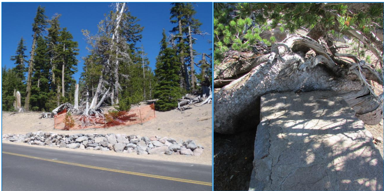
Figure 21. A stone retaining wall was installed to protect a whitebark pine cluster from roadway realignment impacts (left). An old stone wall growing against the bole of a whitebark pine cluster was carefully removed by hand (right). Photos by Jen Beck.
