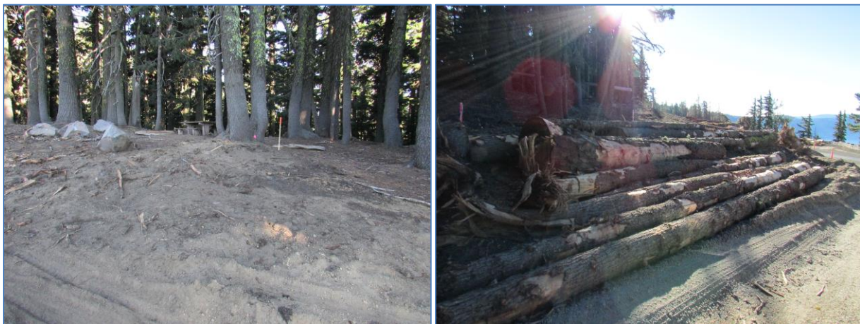
Figure 9. Excessive soil disturbance at the Pumice Point comfort station from driving equipment across slopes (left) and staging downed trees on slopes (right). Photos by Jen Beck.
