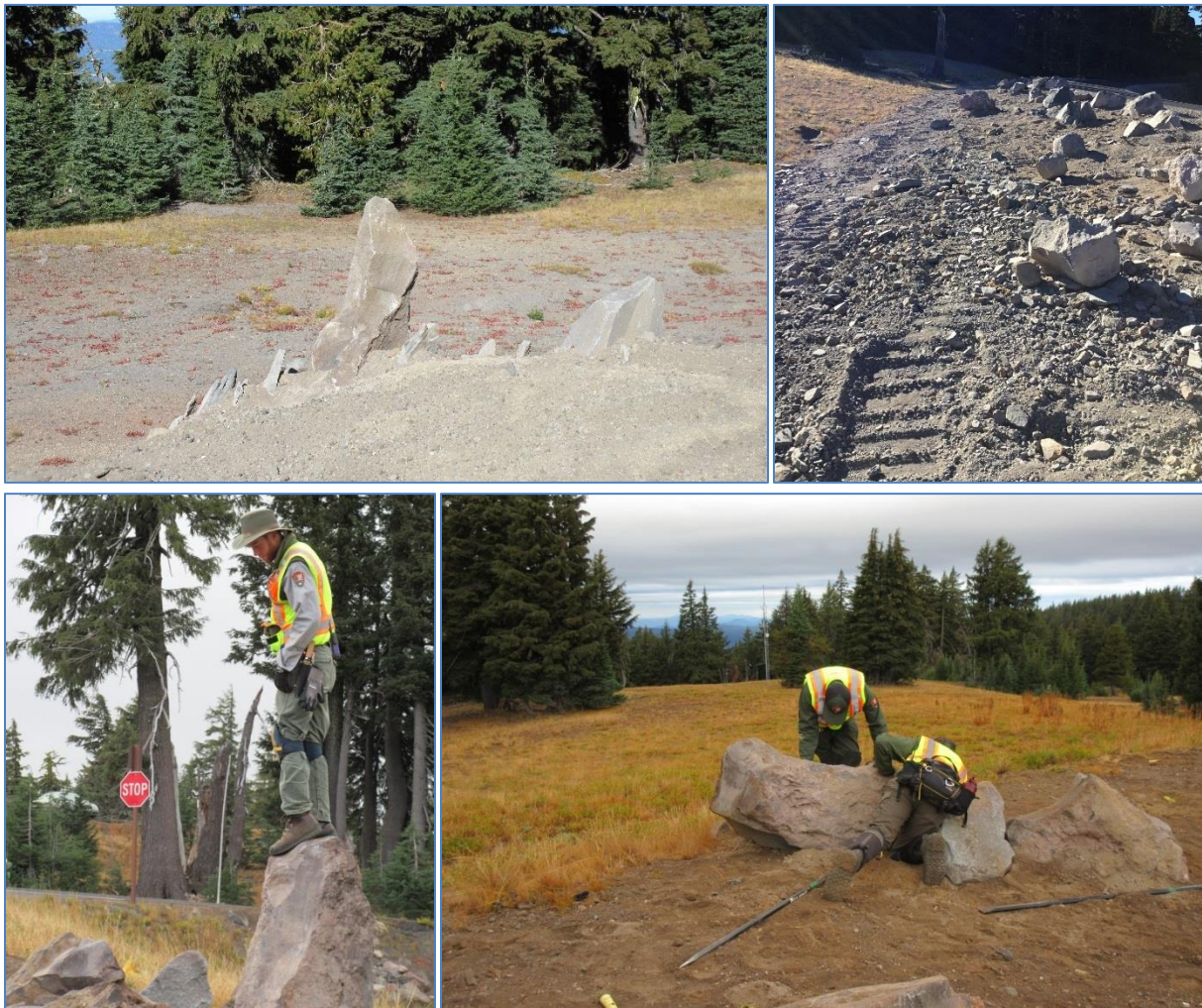
Figure 9. Some sites had boulders placed that did not look natural (top left, bottom left) and/or were left with an excessive amount of gravel at the site (top right). The Botany crew adjusted sites as needed prior to planting/seeding. Photos by Tara Chizinski and Jen Hooke.
