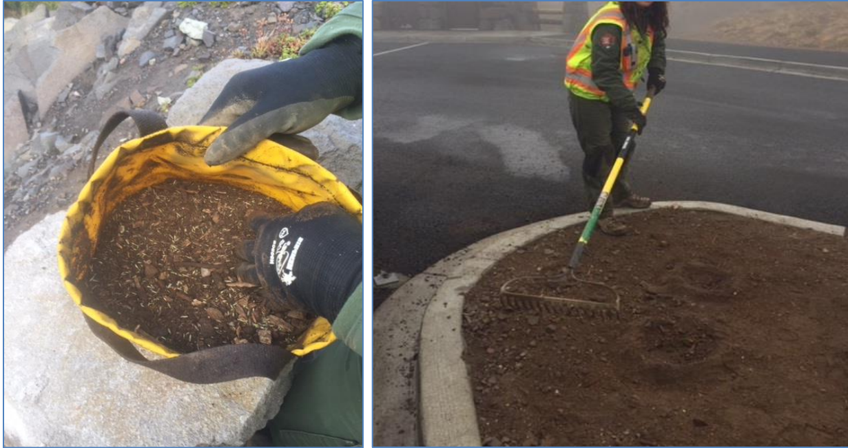
Figure 11. Site specific seed mix (left). Raking seed into a restoration site (right). Photos by Carrie Wyler.
