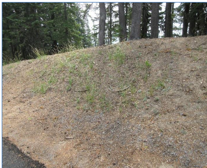
Figure 19. Example of a revegetation site with very good plant establishment after two years. Photo by Carrie Wyler.
