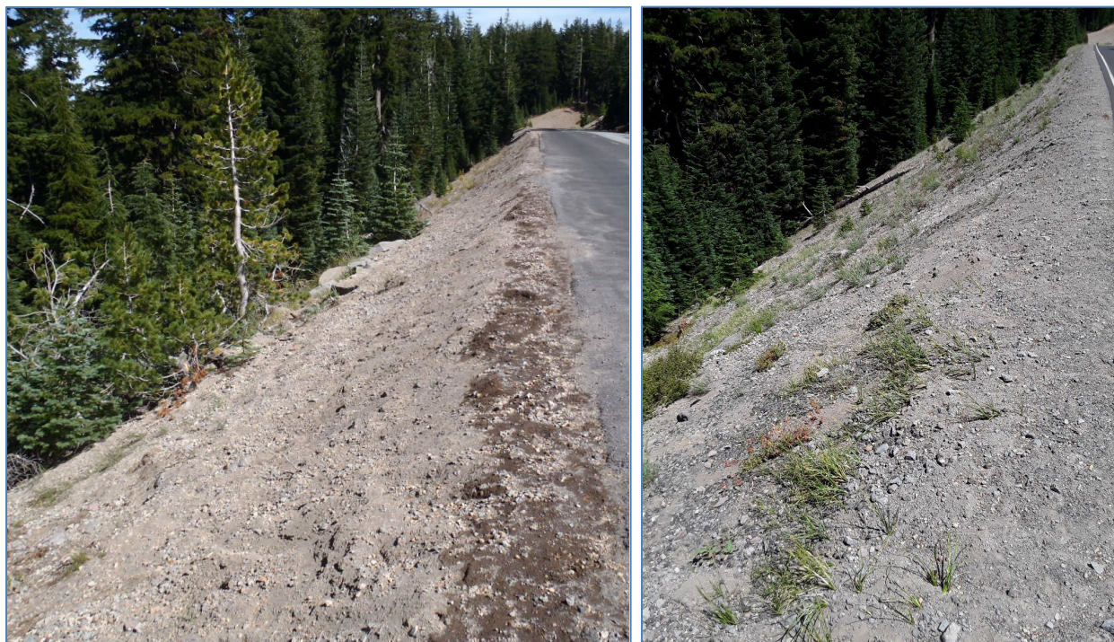
Figure 14. Site NWERD10 in 2016 (left) and in 2021 (right) showing vegetative recovery. Photos by Carrie Wyler.
