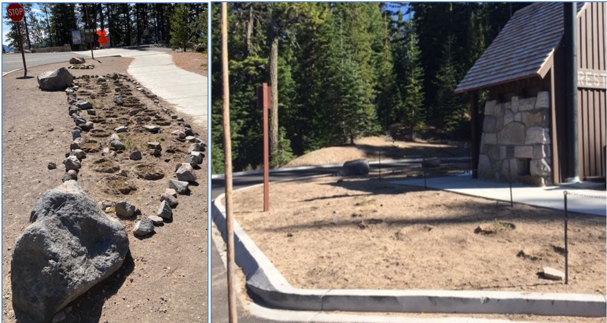
Figure 22. Plantings in groups with rock borders to mitigate trampling in heavily trafficked Cleetwood Cove parking lot areas (left). The area at the back of the Cleetwood Cove parking lot will be adjusted to allow for RVs to drive around the comfort station (right). Photos by Carrie Wyler.
