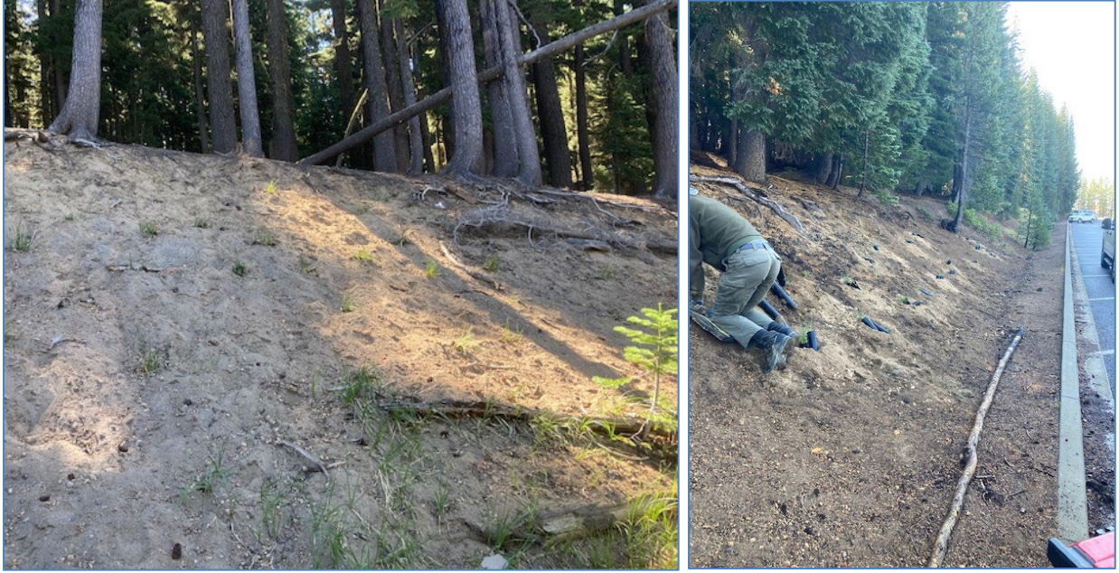
Figure 24. The steep slope of the embankment in the Cleetwood Cove parking lot with Hall's sedge taking hold (left). Planting more Hall's sedge on the embankment in 2022 (right). Photos by Carrie Wyler.
