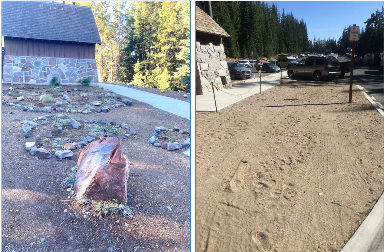
Figure 23. Plantings in groups with rock borders to mitigate trampling in heavily trafficked Cleetwood Cove parking lot areas (left). The area at the back of the Cleetwood Cove parking lot needs to be adjusted to allow for RVs to drive around the comfort station without damaging the landscaping island (right). Photos by Carrie Wyler.
