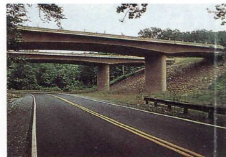
Approach Bridges/Tenn. Portal
