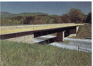
CSX Railroad Bridge
