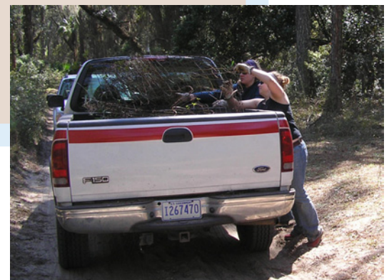
Students removed 6 miles of fencing from designated Wilderness
