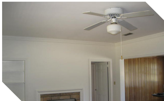
White Cottage has been painted and repaired.
