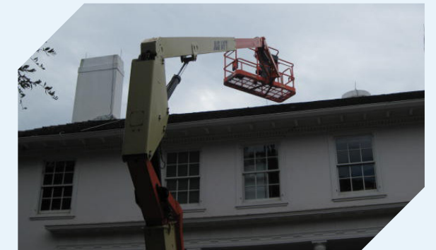
Employee Mickey Bosworth working on the roof at Plum Orchard.
